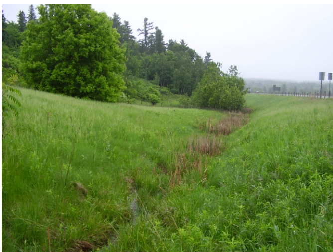
← Photo 6 Drainage ditch flanking the east side of the highway between Culverts 2 and 3. Photo taken facing south.
