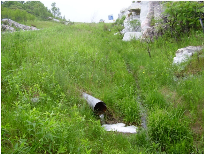
← Photo 4 Photo showing Culvert 3 discharging water into the drainage ditch on the east side of Highway 17 which then flows to the south of the site and into Culvert 2. Photo taken facing north.
