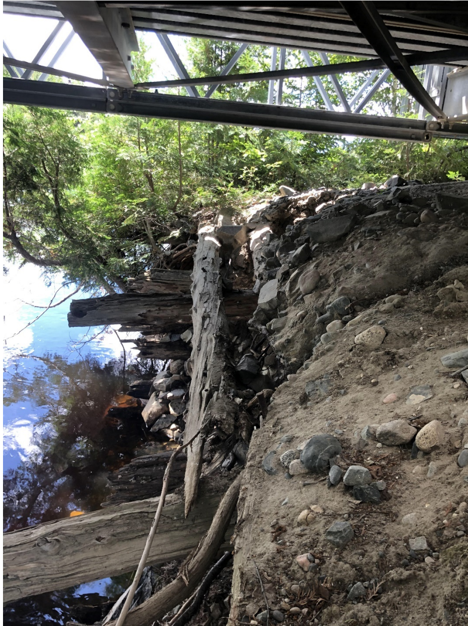
Photo 4: North abutment, forward slope and timber cribs.
