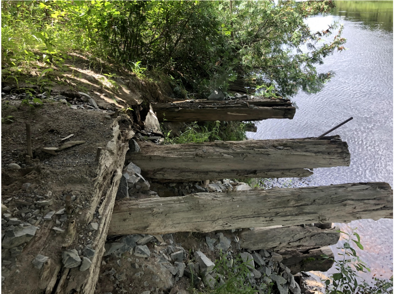
Photo 4: South Abutment, existing timber cribs
