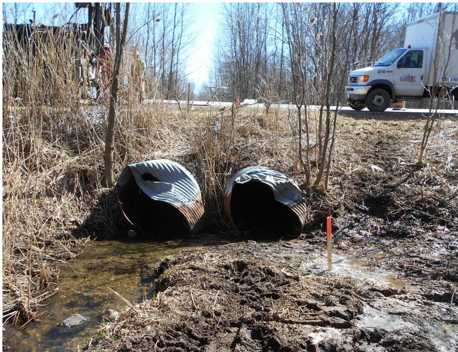
Figure 5: Existing condition of culverts and embankment at inlet
