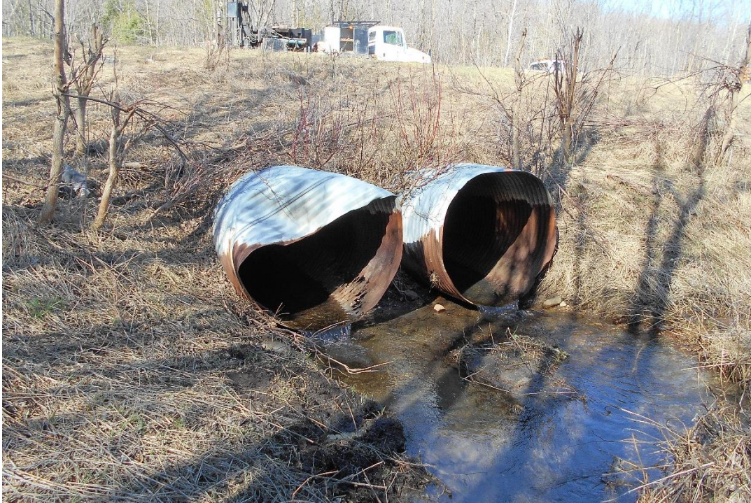
Figure 3: Existing condition of culverts and embankment at outlet
