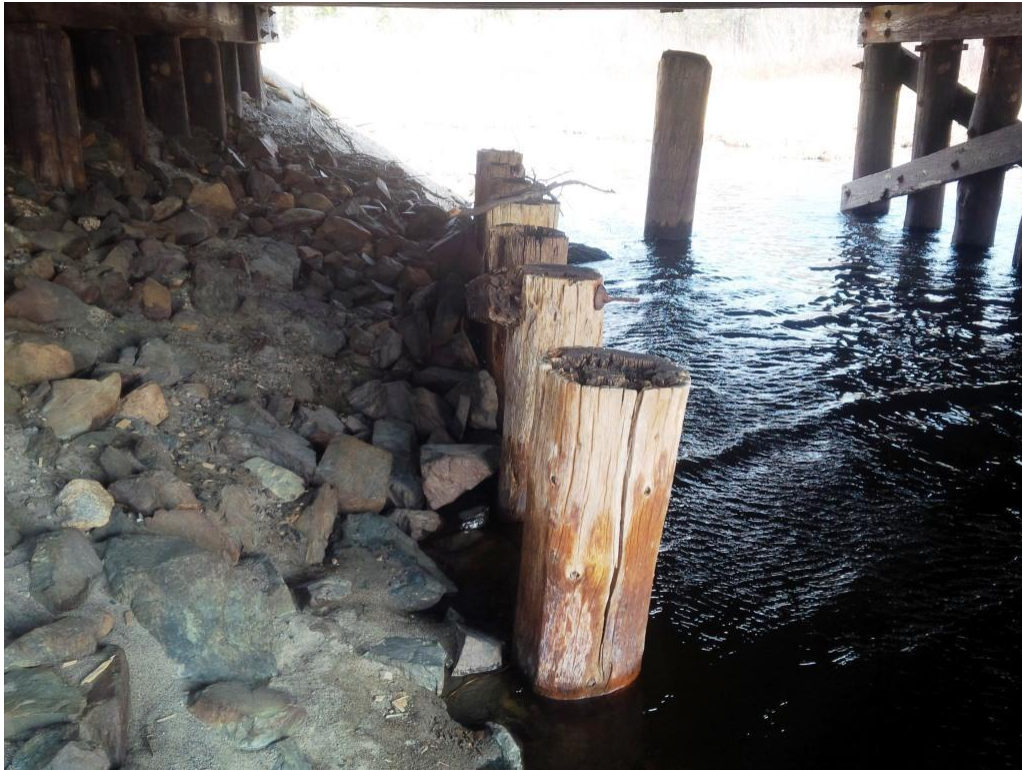
Photo 9 - North Abutment –Front Slope and Existing Cut-off Piles
