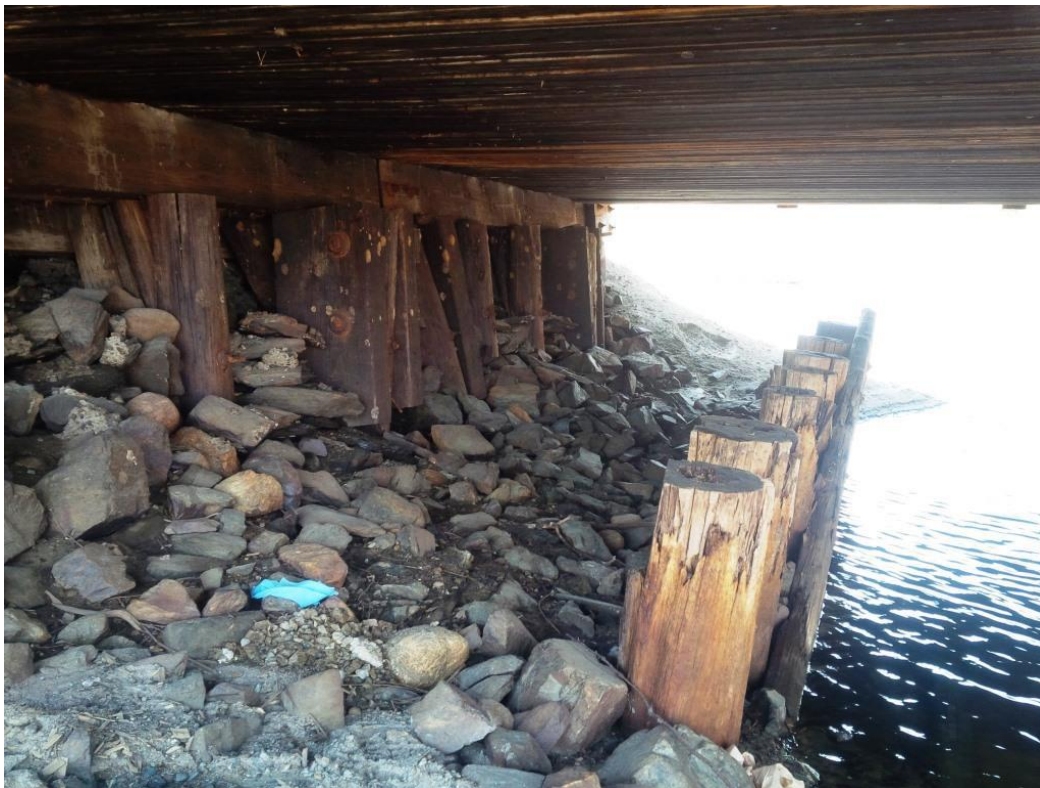
Photo 10 - South Abutment - Front Slope and existing cut-off piles
