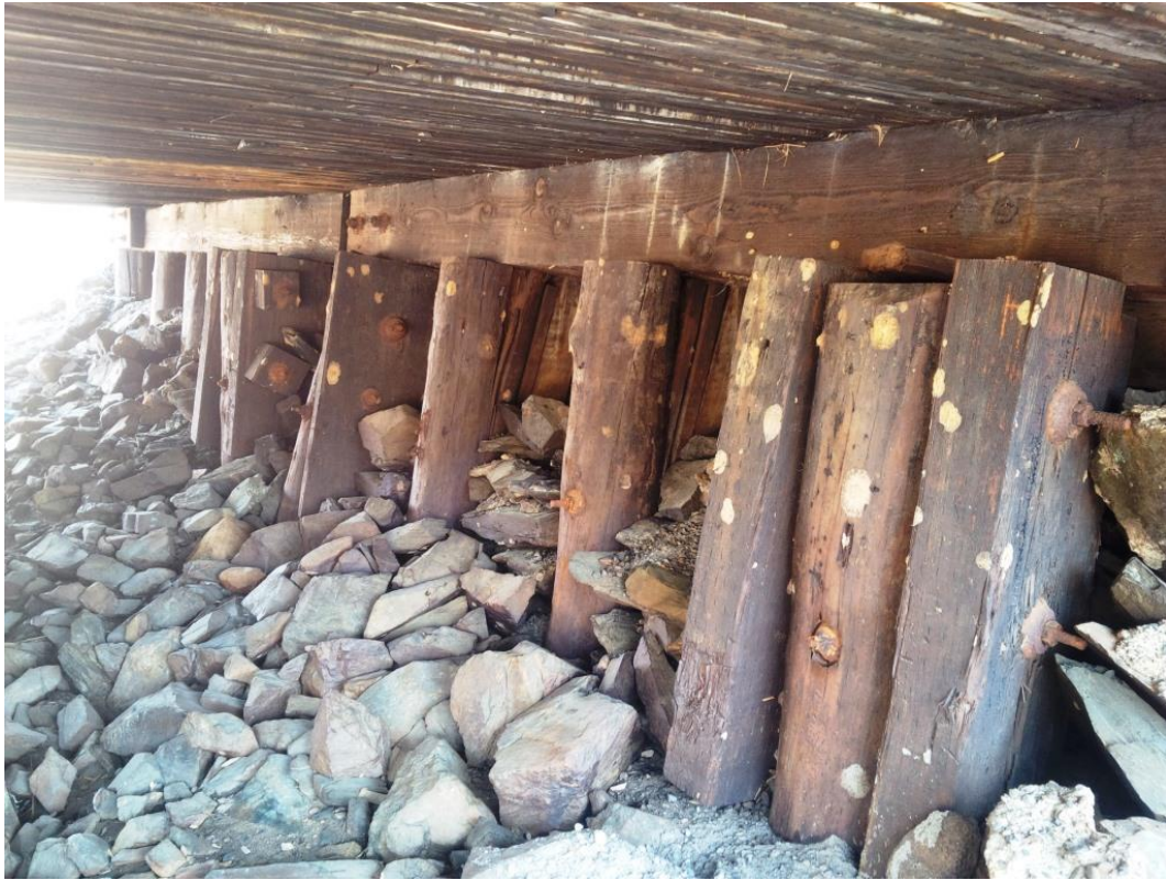
Photo 7 - South Abutment Piles – Looking West
