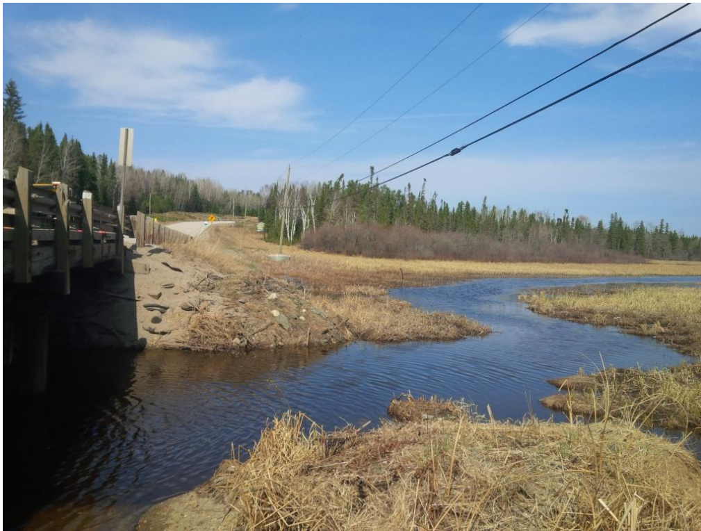
Photo 12 - Looking North from SE corner – Noticeable Highway 72 Embankment Sag
