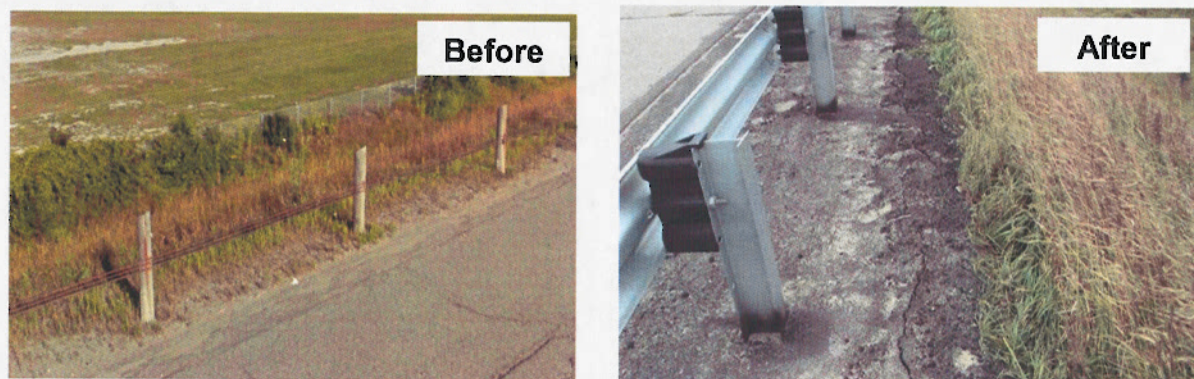
Figure 3: Before and After Steel Beam Guide Rail and Asphalt Shoulder Treatment Installation
