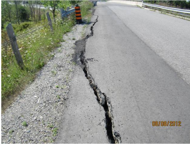
Figure 2: Tension crack at the edge of pavement
