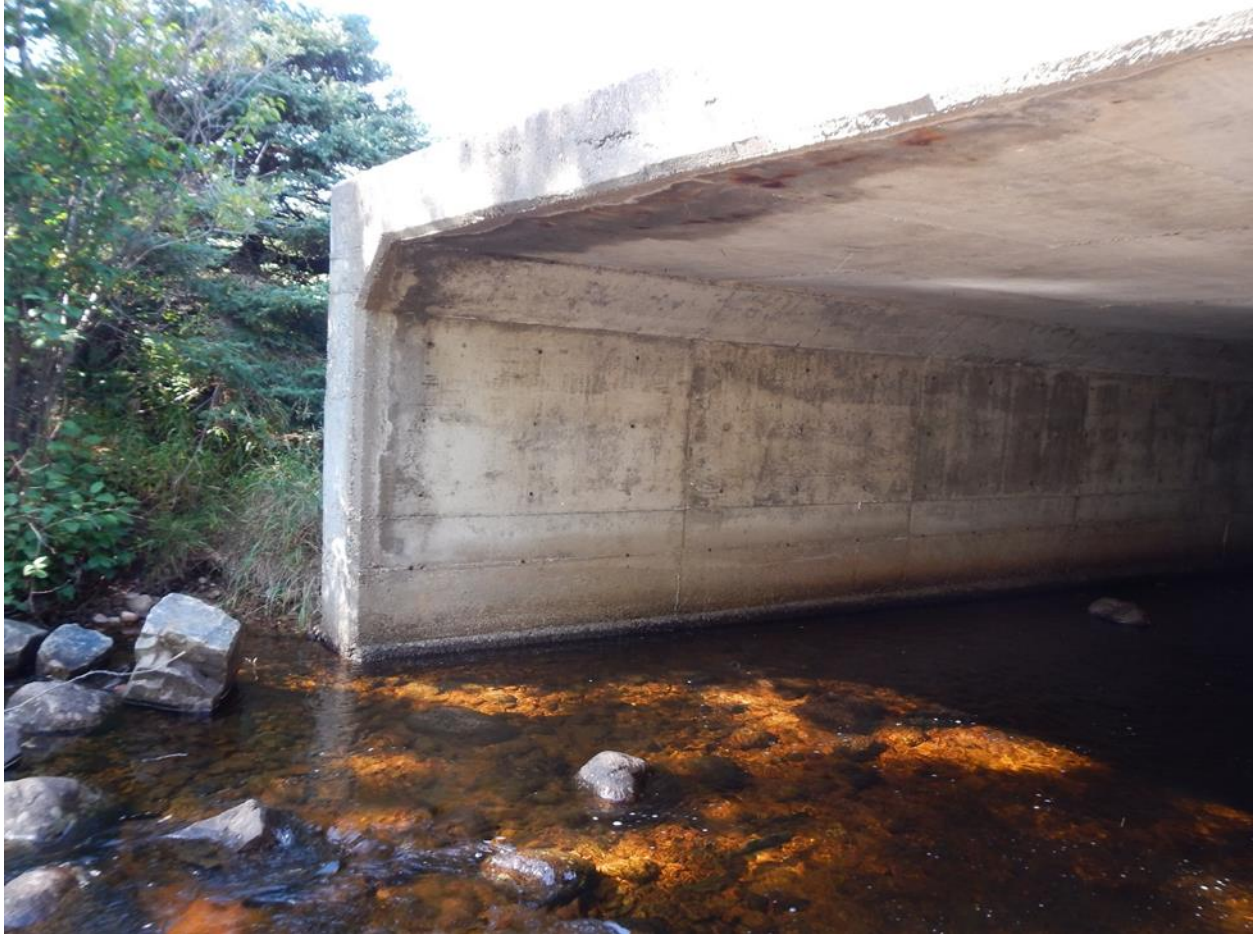
Photo 4: Culvert outlet looking north, showing delamination of soffit and scaling and spalling of lower wall (June 14, 2013)
