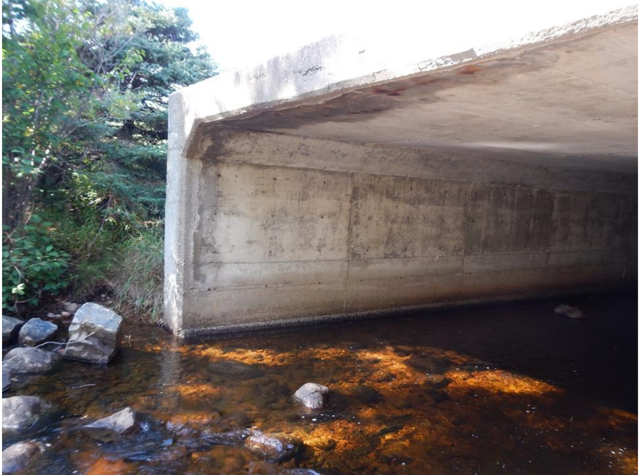
Photo 5: Culvert outlet looking north, showing delamination of soffit and scaling and spalling of lower wall (June 14, 2013)
