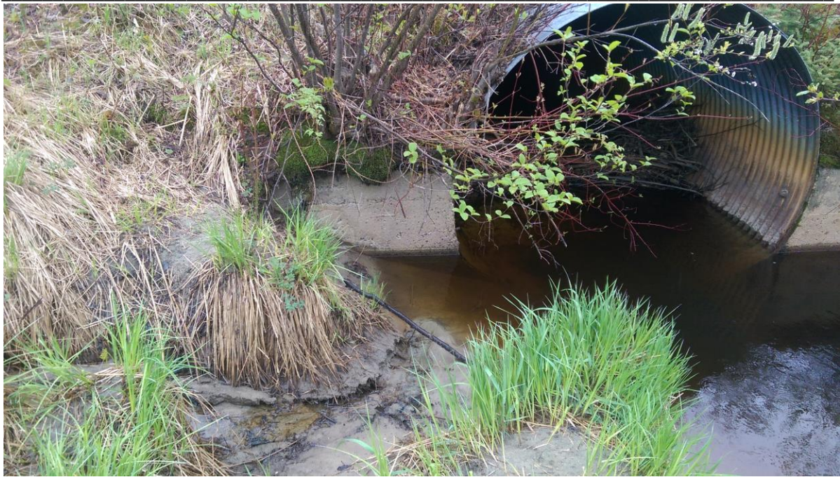
Photo 3: Erosion of Watercourse at North East Inlet
