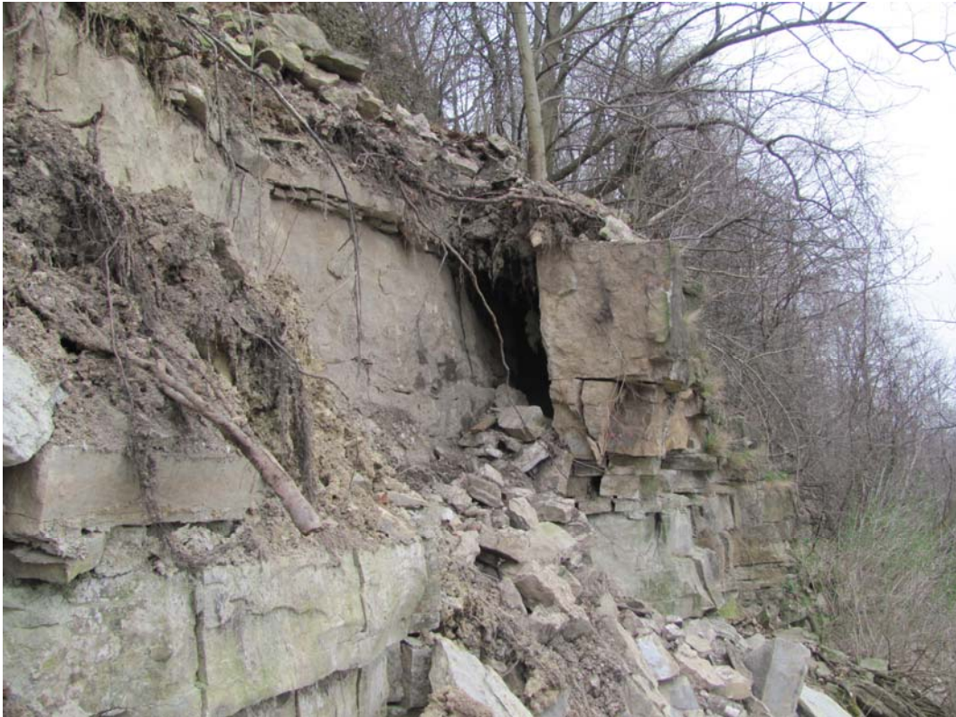
Image 3. Void to right of source area in Image 2, isolates approximately 7 cubic metres of loose rock. Approximate total rock to be removed in this area is 15 cubic metres.
