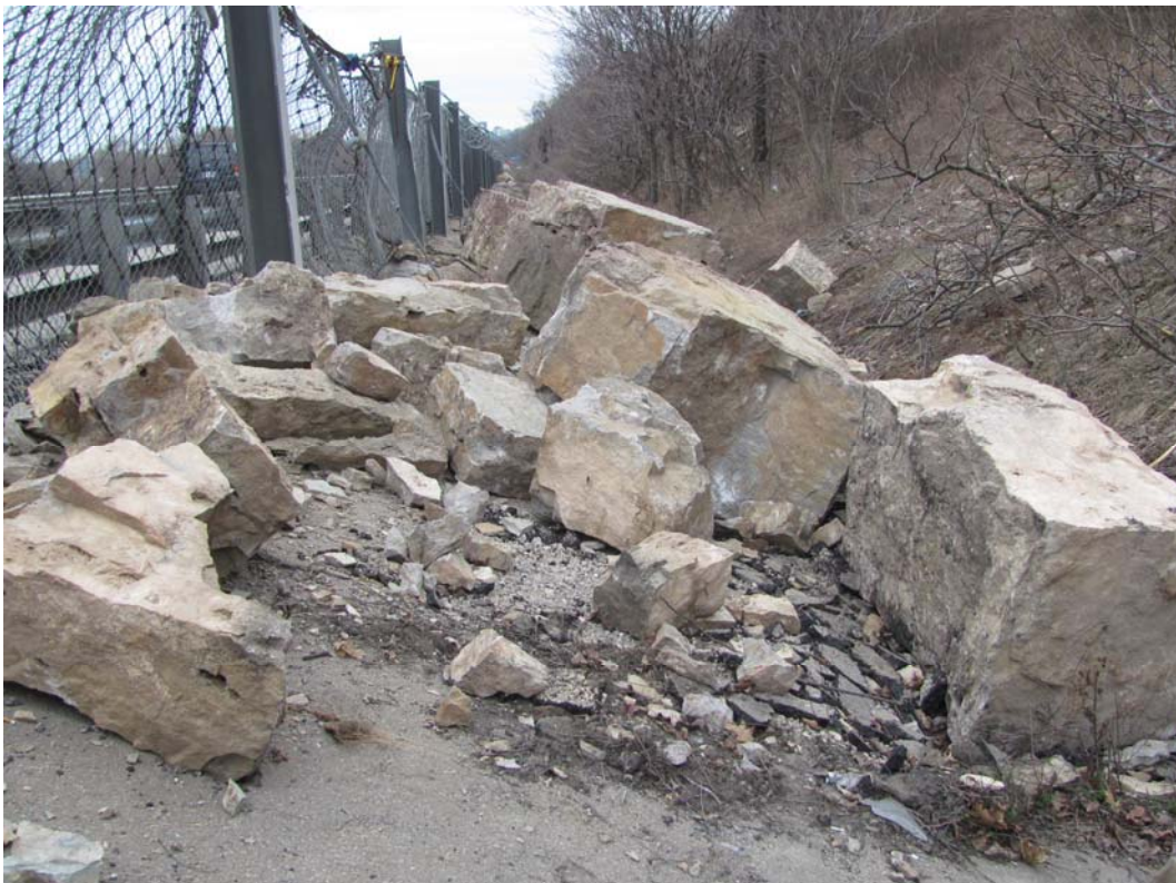
Image 6. Accumulated rockfall material from main event, 13 March 2012. (Image date – 29 March 2012)
