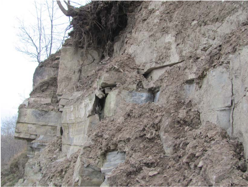
Image 11. Close-up of crest of failed area, upper left in Image 9. (Image date – 29 March 2012)
