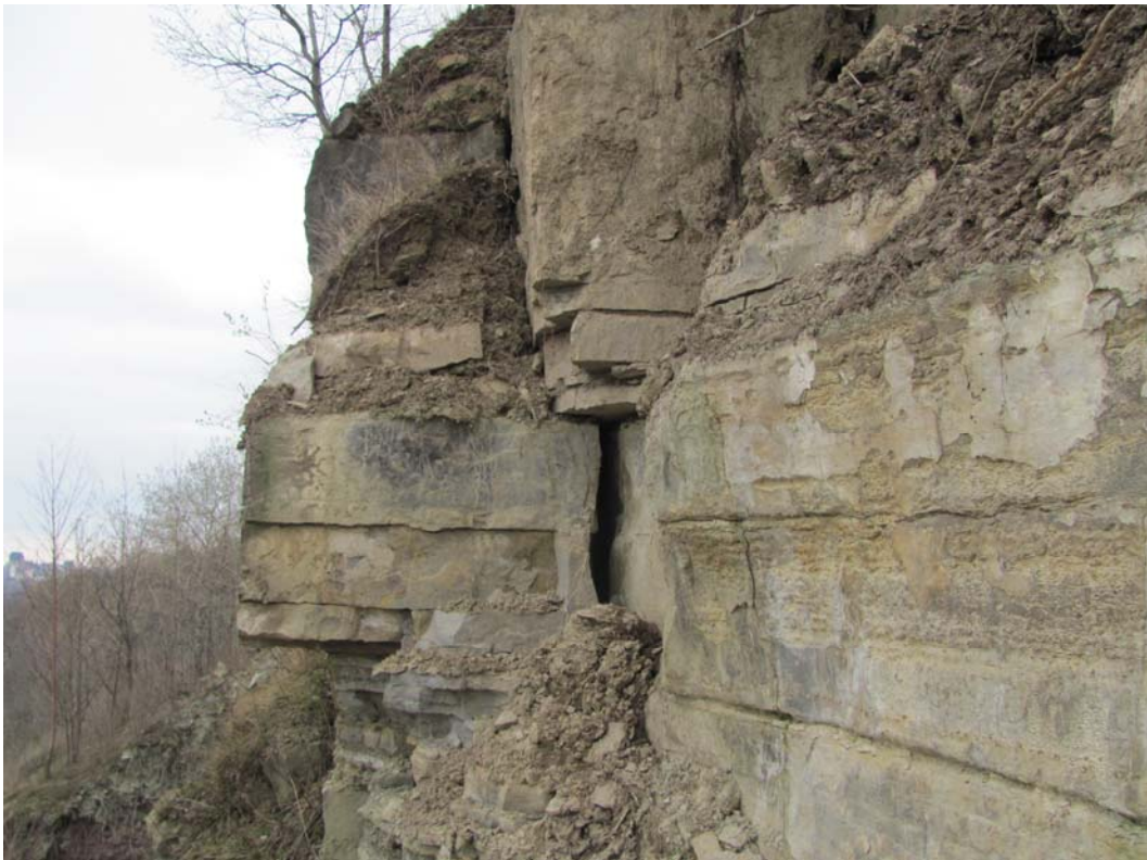
Image 12. Typical crest conditions in rock formation that failed, adjacent to second event. (Image date – 29 March 2012)
