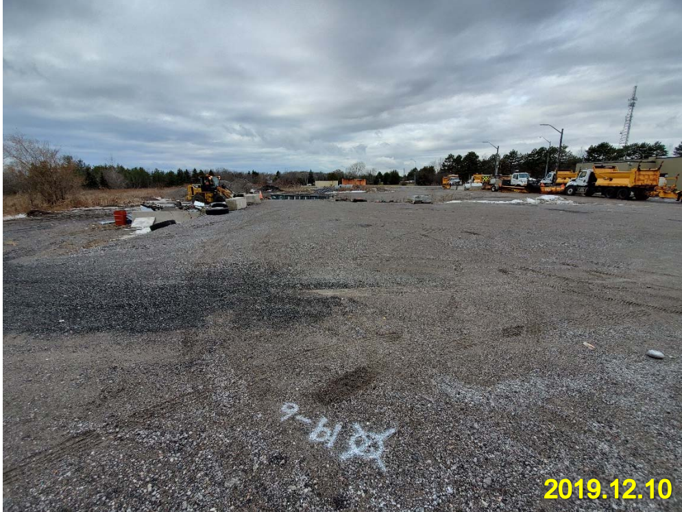
Photo 1. Looking west from BH 19-6 towards proposed garage building
