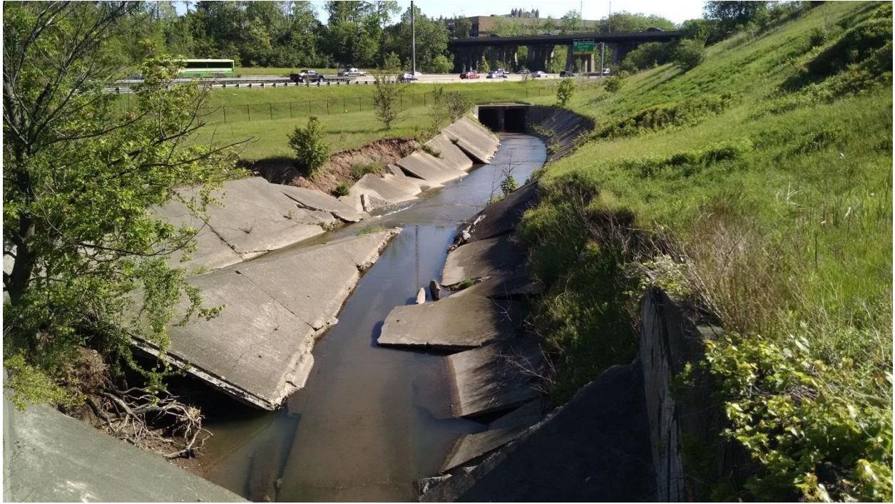
Photograph 15 – Failed channel looking northeast from municipal drain outlet
