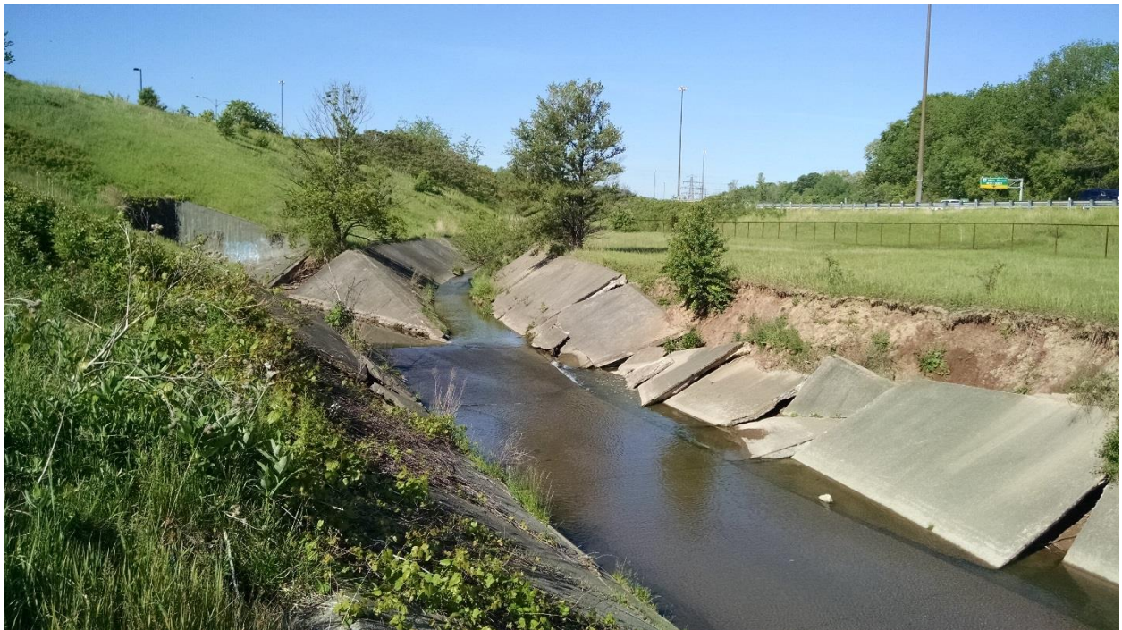
Photograph 16 – Failed channel looking west towards municipal drain outlet on left
