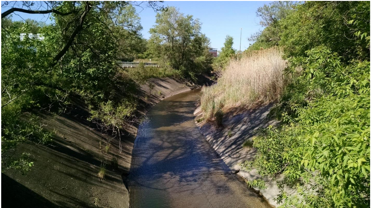
Photograph 24 – Channel looking west from inlet to culvert under Main Street West. Note wet area on right side of channel.
