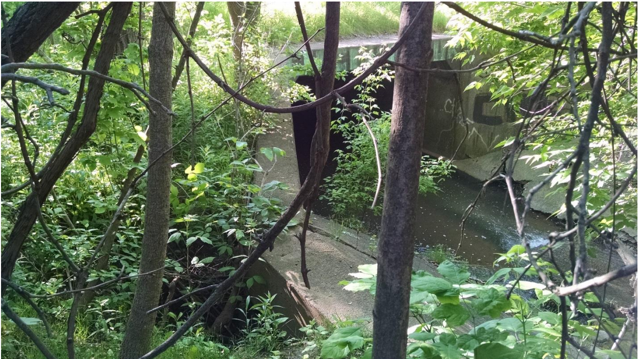
Photograph 8 – Inlet to culvert under ramp from Main Street to Highway 403 east. Note void behind wingwall.
