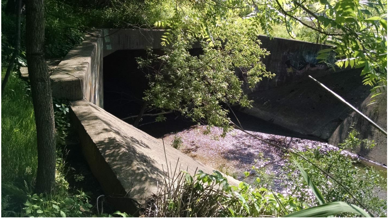
Photograph 23 – Inlet to culvert under Main Street West. Note void behind channel lining.
