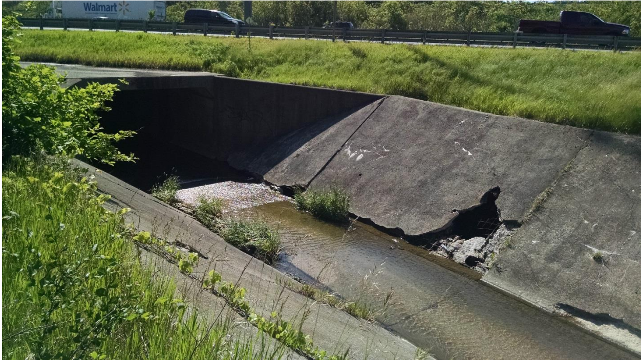
Photograph 11 – Inlet to culvert under Highway 403 east of Aberdeen Avenue. Note void under lining.
