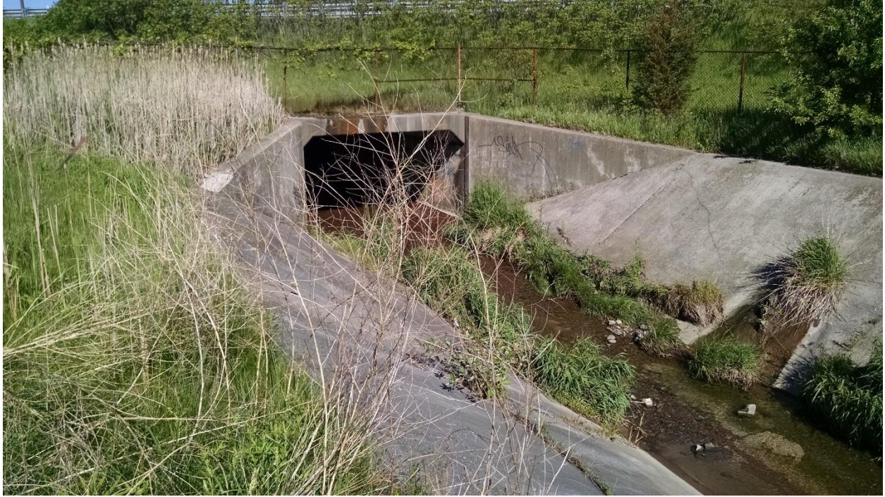
Photograph 13 – Culvert outlet on south side of Highway 403 between Aberdeen Avenue and Longwood Road. Note wet ground behind wingwall (upper left of photo) and seepage on top of culvert.
