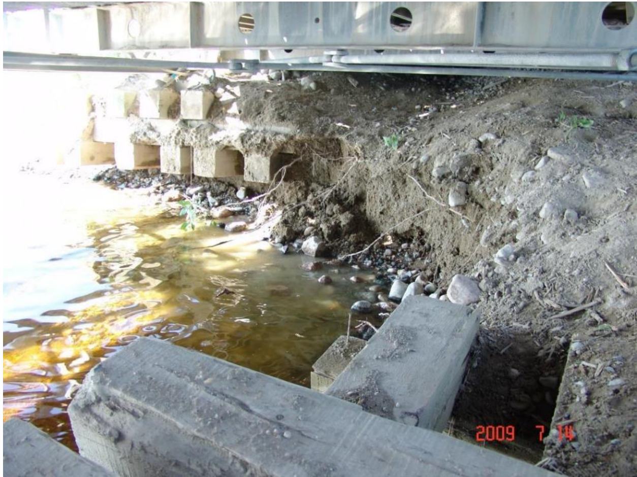
Photo C3: Erosion at west abutment foundation (Date taken: July 7, 2009; provided by MTO).
