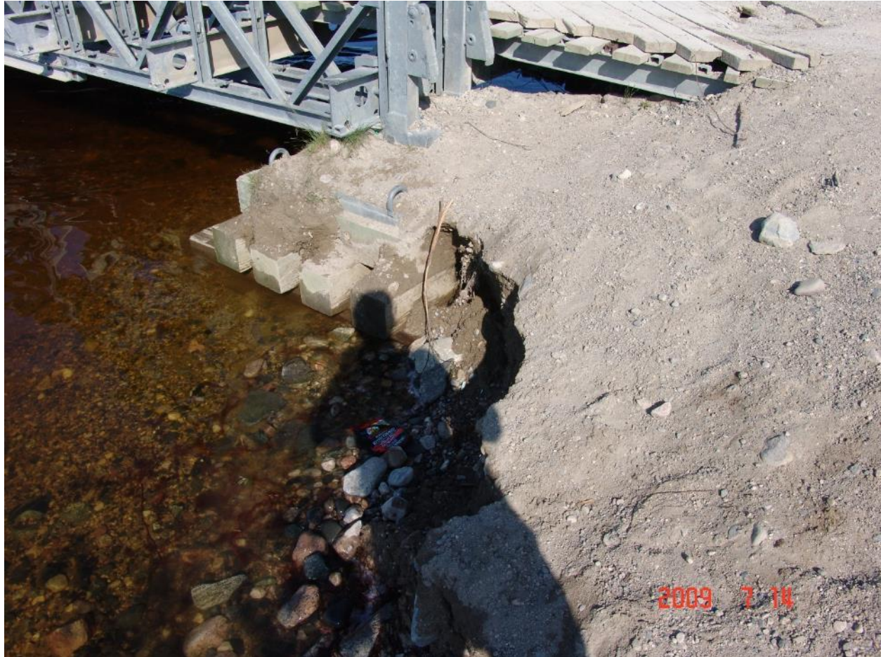
Photo C4: Erosion at east abutment foundation (Date taken: July 7, 2009; provided by MTO).
