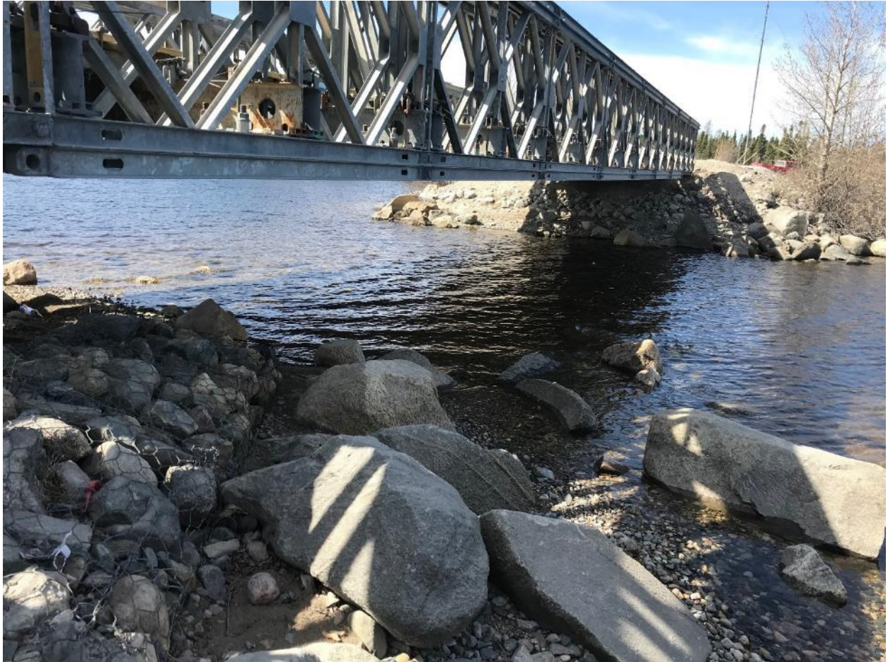
Photo C13: North side of bridge looking west showing large boulders and gabion baskets for erosion protection (Date taken: June 4, 2019).
