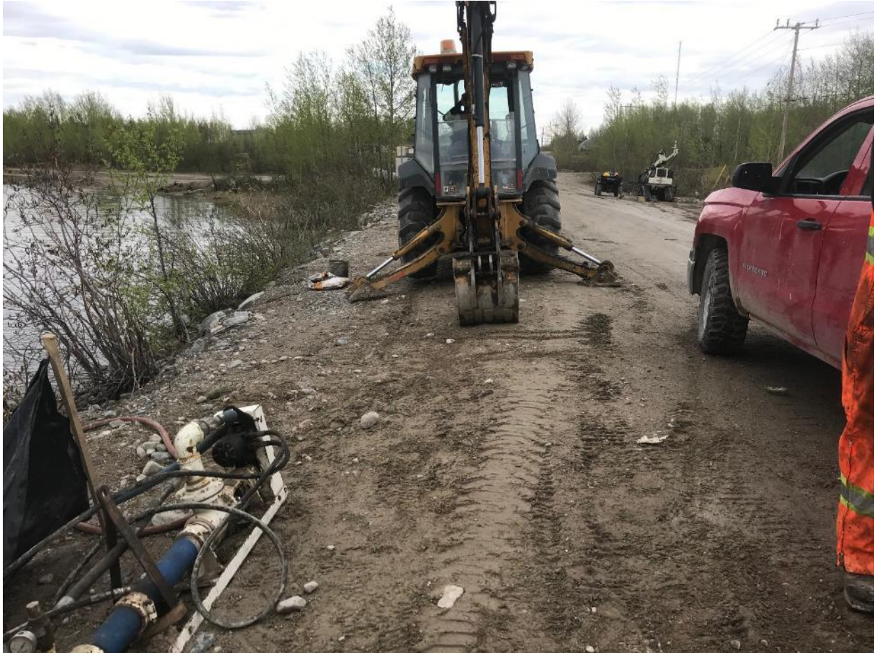
Photo C7: Backhoe at Test Pit TP-02 on north side of east approach embankment, looking east (Date taken: June 8, 2019).
