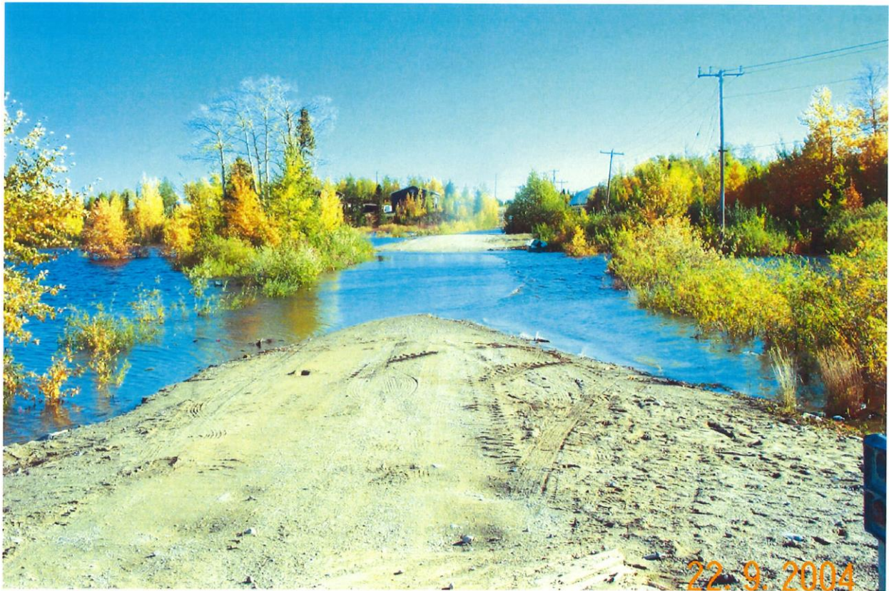
Photo C2: Overtopping of east causeway embankment (Date taken: Sept. 22, 2004; provided by MTO).
