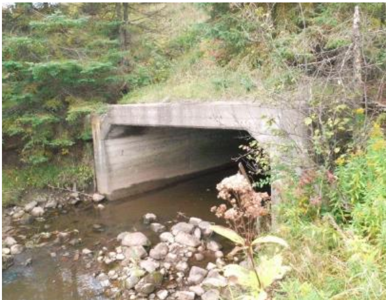
Photograph 4: Culvert Outlet
