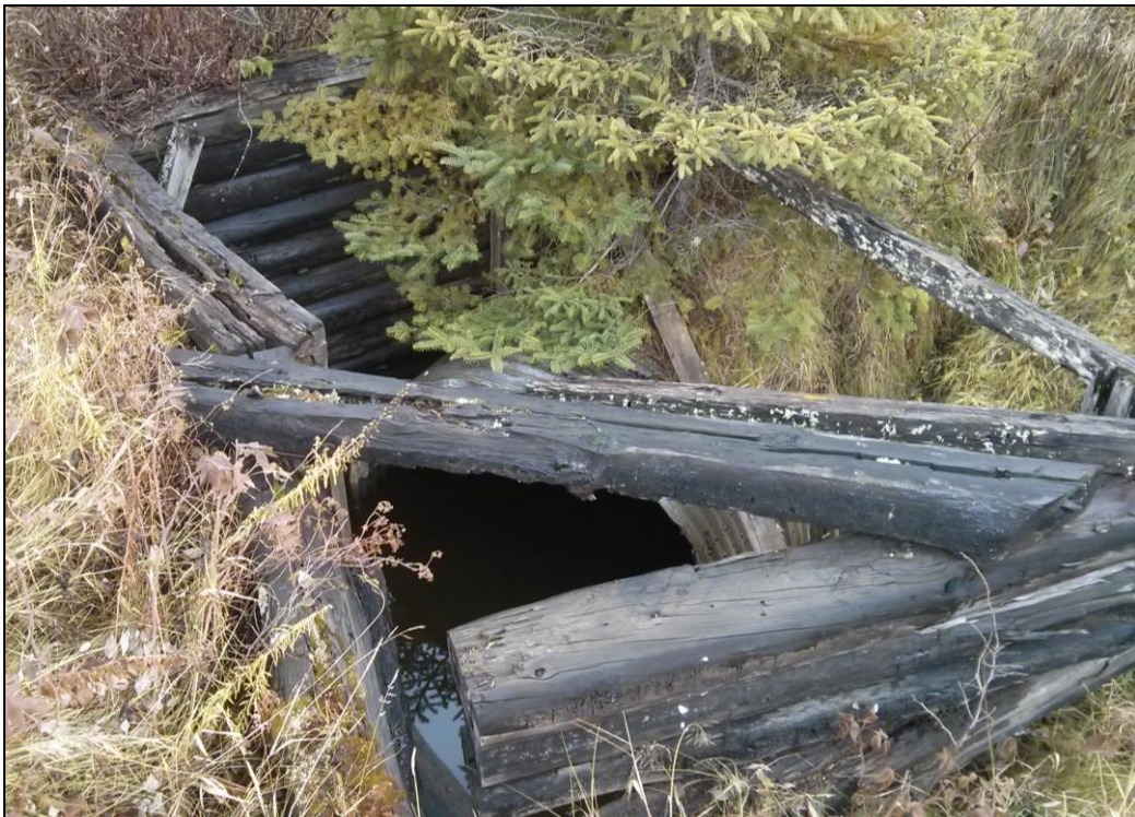
Photograph 8: Existing Itzcaulde Creek culvert Inlet.
