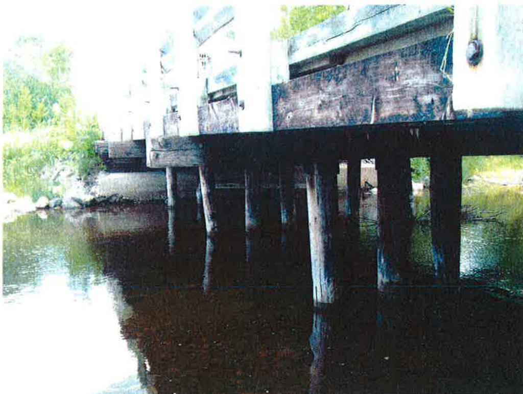
Photograph D3. Existing Harmony Beach Road Bridge Foundations
