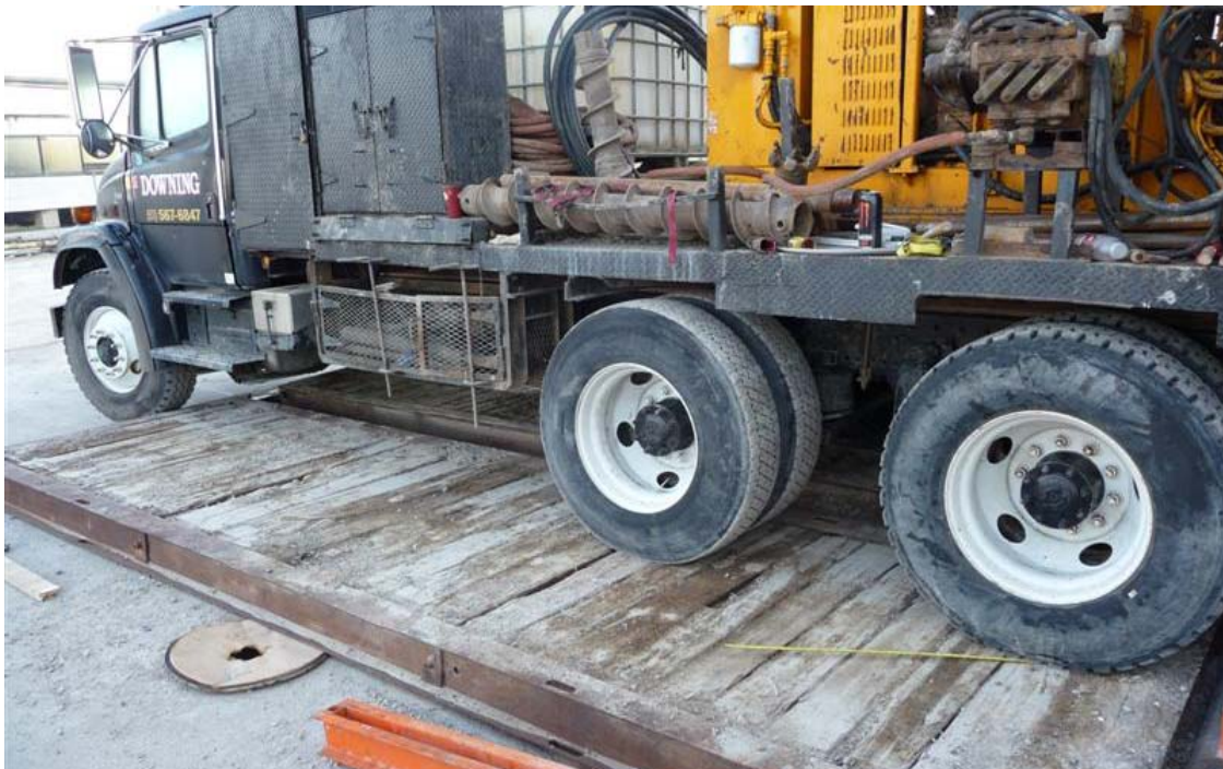
Figure 2 – Temporary mats for the drill rig to bridge voids under the asphalt
