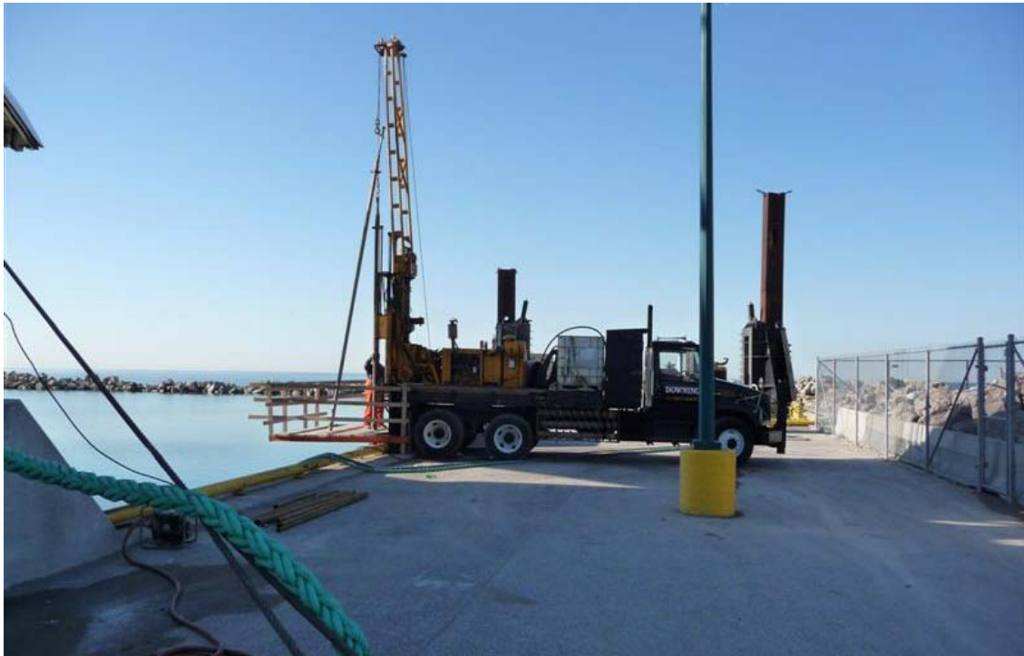
Figure 1 – Drill rig and temporary platform over Lake Erie (09-03)
