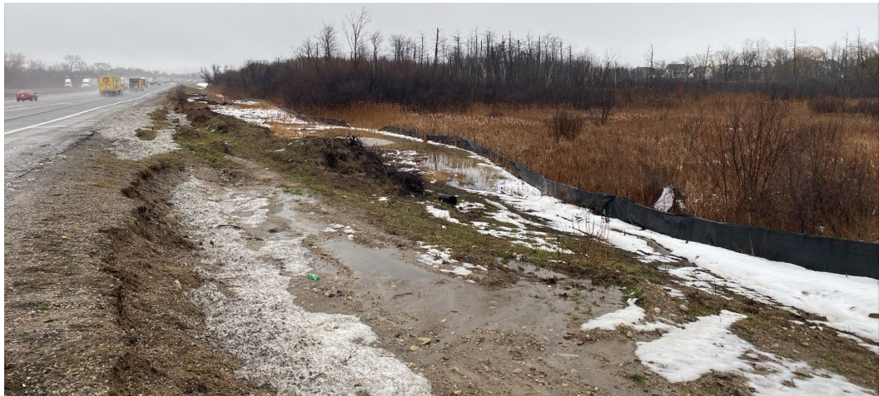
Figure 2.1: Slumping of highway embankment slope, visible new fill to the left, visible surface water on peat bog - View of the site looking east
