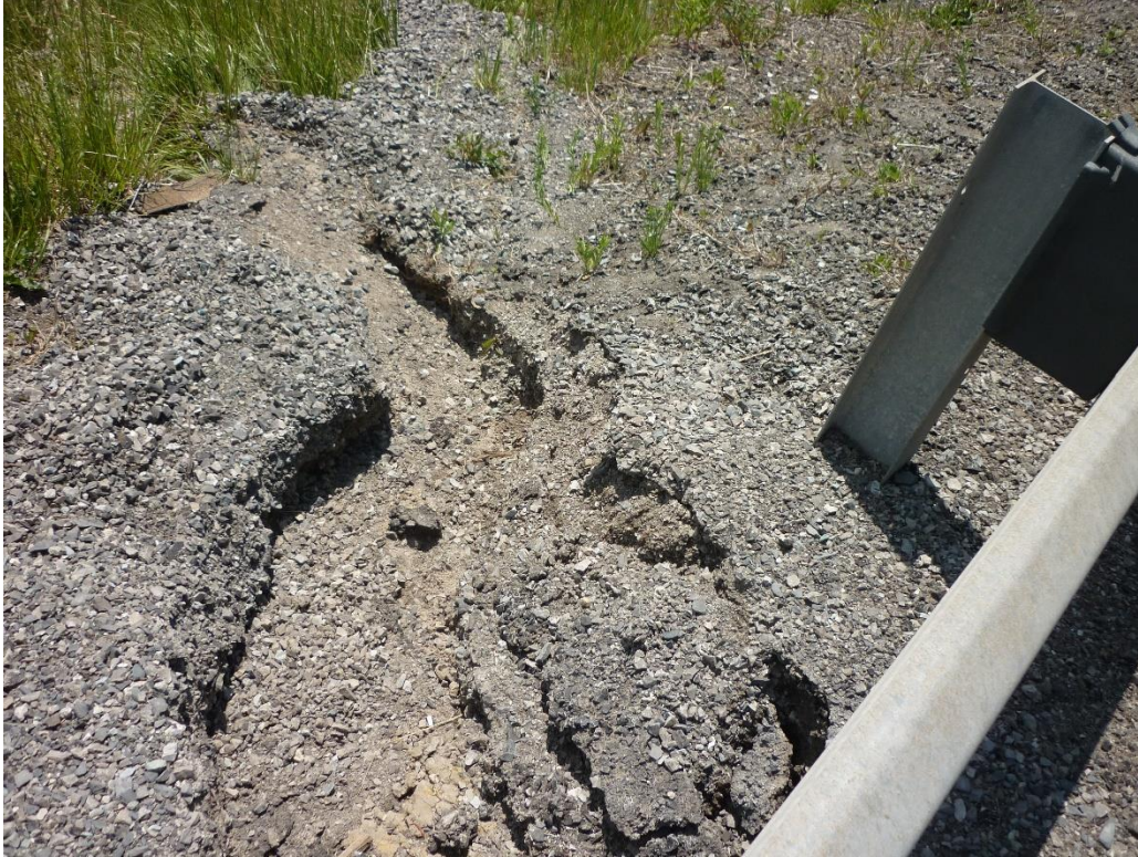
Photo 5 Gully at Slope Crest (east side)
