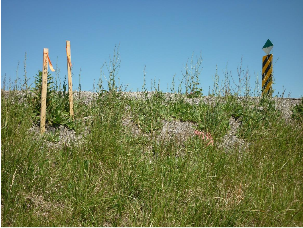
Photo 1 Sloughed Granular Materials on Upper Slope near Station 15+300 (east side)
