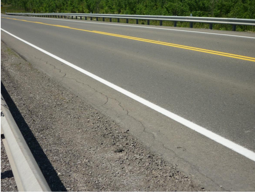
Photo 3 Asphalt Cracks on Road Shoulder near Station 15+500 (east side)
