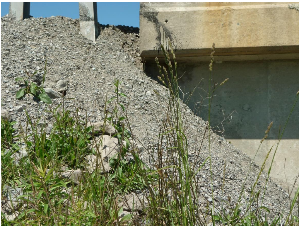
Photo 2 Over-Steepened Slope at South Abutment (east side)
