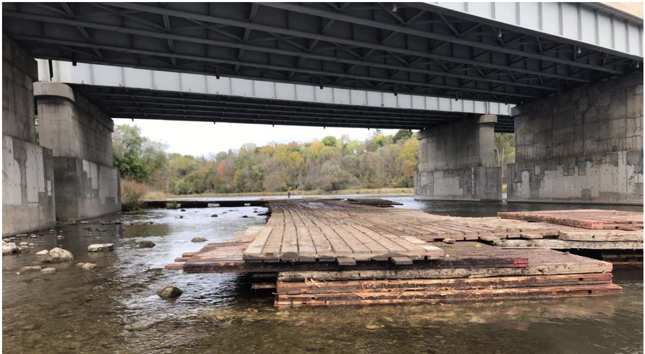
Photograph 8 – Access mats for Pier 2 drilling, facing north
