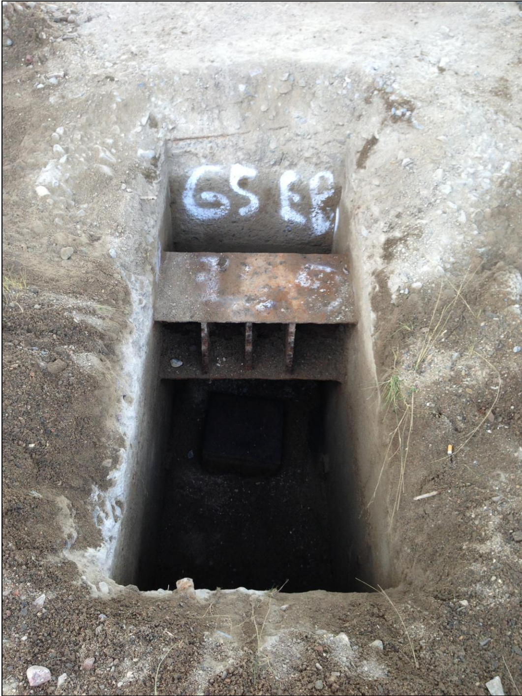
Photograph C1 – Pile Cap Cut-out and Reaction Beam at Pier G-5
