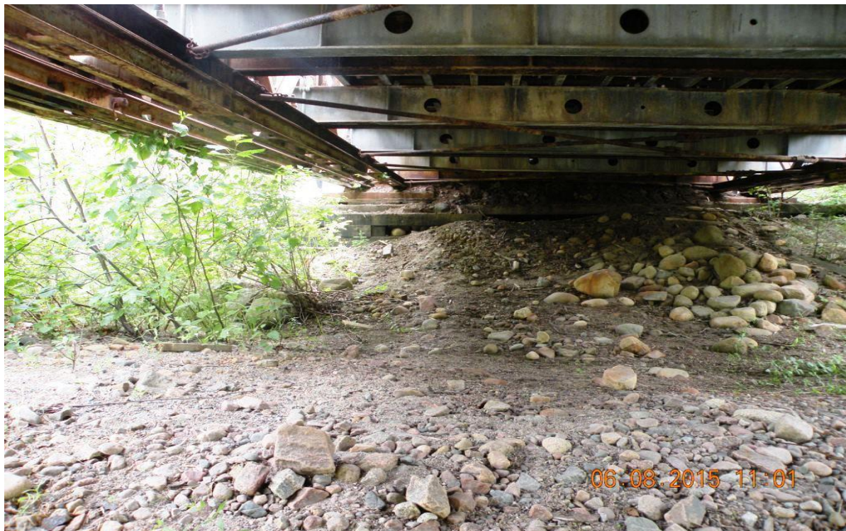
Photograph 3 – East abutment and view of timber crib
