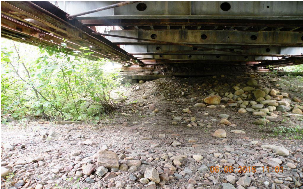
Photograph 3 – East abutment and view of timber crib
