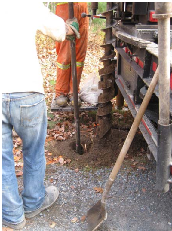
Photograph 7: MMM11-02 borehole drilling (Nov.2, 2011).
