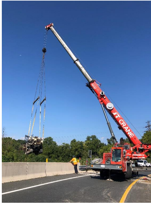
Photograph 13. Crane lifting Geoprobe for EXP-BH15 (looking northwest), September 5, 2023
