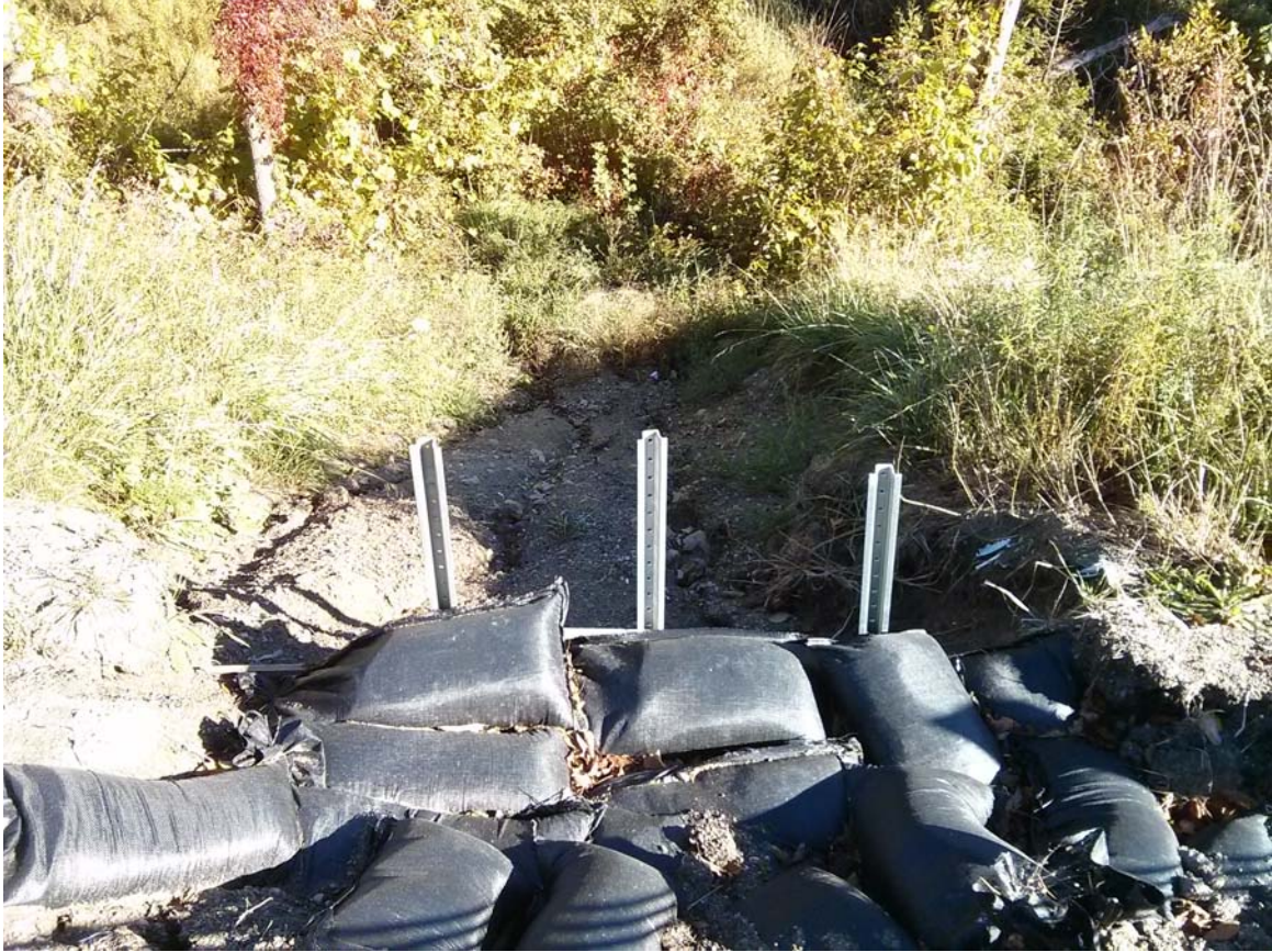
Photo 3: Looking Northward (perpendicular to Highway) from westbound shoulder showing sandbags and erosion gullies along slope failure on north side of highway
