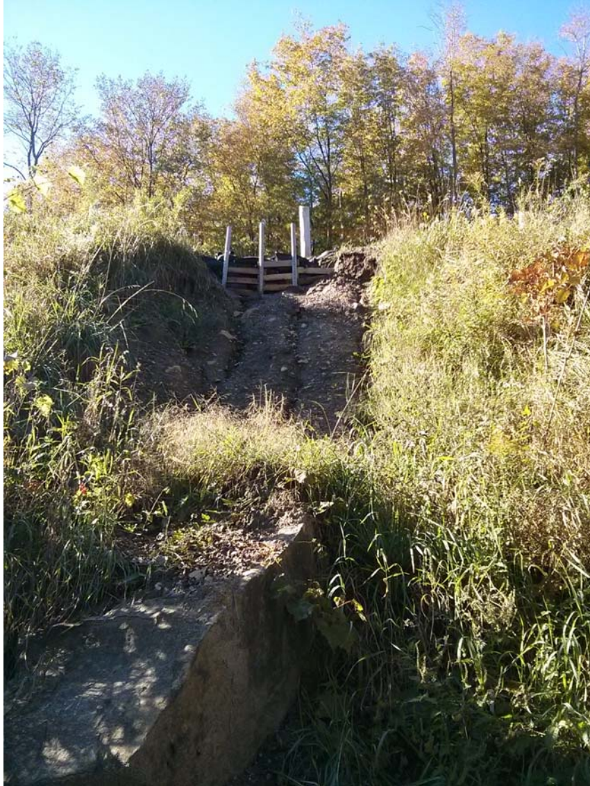
Photo 4: Looking Southward (toward Highway) from north toe of slope showing erosion gullies and soil deposition along slope failure on north side of highway
