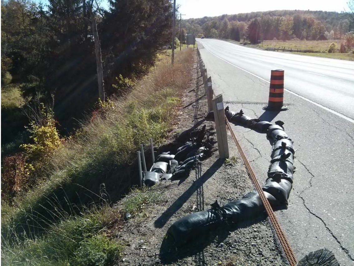
Photo 2: Looking Eastward (toward Owen Sound) from westbound shoulder showing pylons and sandbags outlining slope failure on north side of highway. Also note longitudinal cracking on shoulder parallel to highway.
