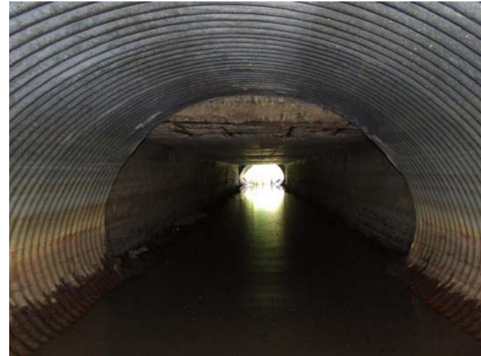
C03 - Station 12+352 - Culvert Extension and Original Concrete culvert
