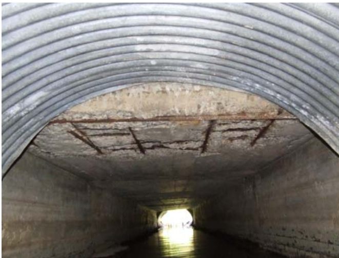
C03 - Station 12+352 - Culvert Extension and Original Concrete culvert
