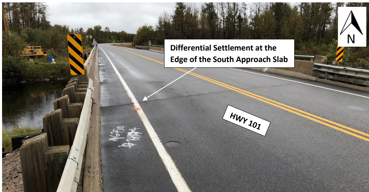
Photo C1-2: Looking towards North of Highway 101 – Differential Settlement at the Edge of South Approach Slab (September 2018)
