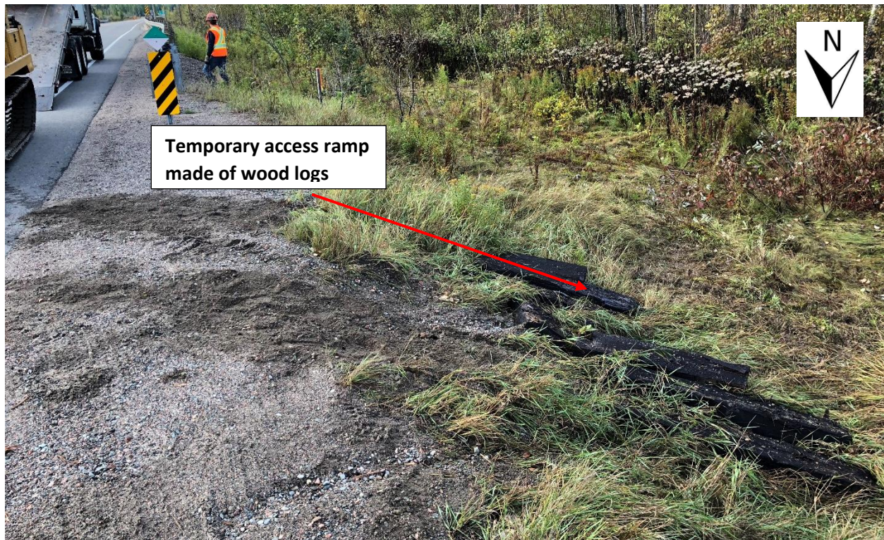
Photo C2-7: Looking Southwest – Showing temporary access ramp constructed of wood logs (September 2018)
