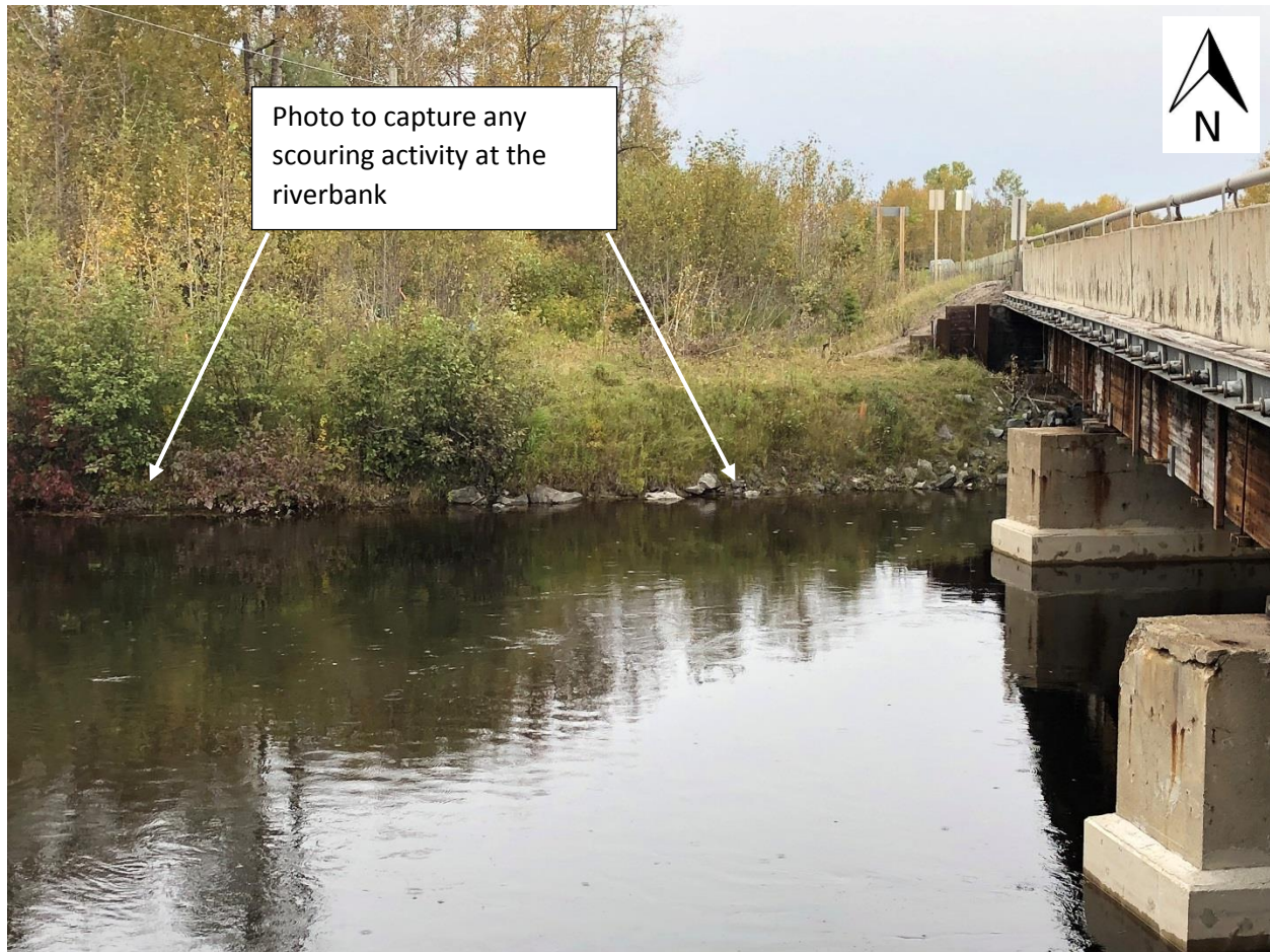
Photo C1-5: Looking towards North at the river bank for erosion activity at the north abutment along the proposed bridge alignment (September 2018)
