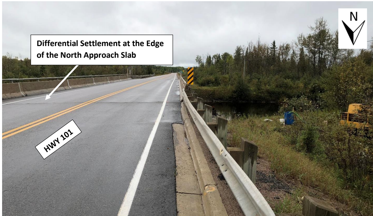
Photo C1-3: Looking towards South of Highway 101 – Differential Settlement at the Edge of the North Approach Slab (September 2018)
