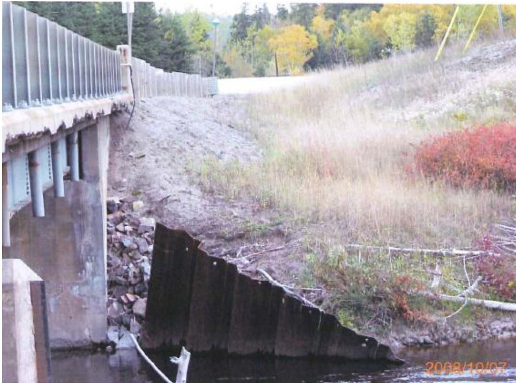
West Abutment north side (failed sheet piling)
