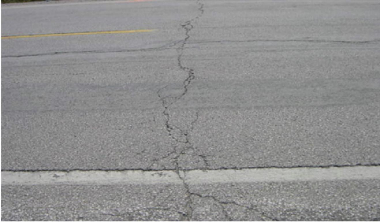
STA 16+967 - transverse crack on pavement above Culvert C4 looking east
