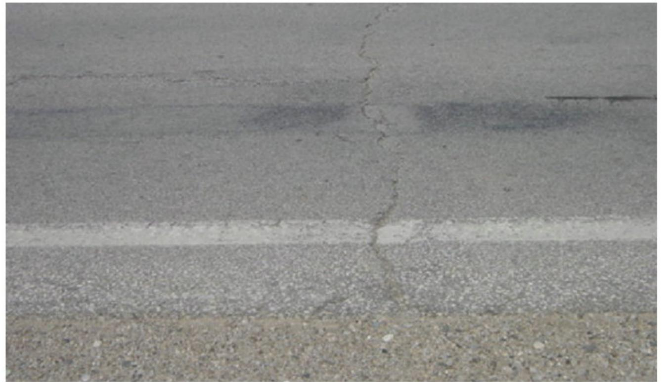
STA 16+967 - transverse crack on pavement above Culvert C4 looking west
