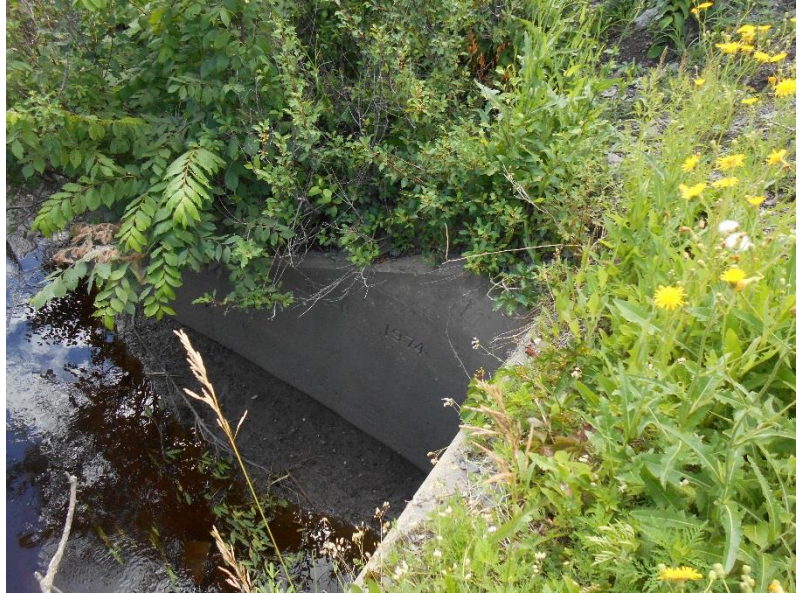
Condition of south tapered portal wall at inlet
