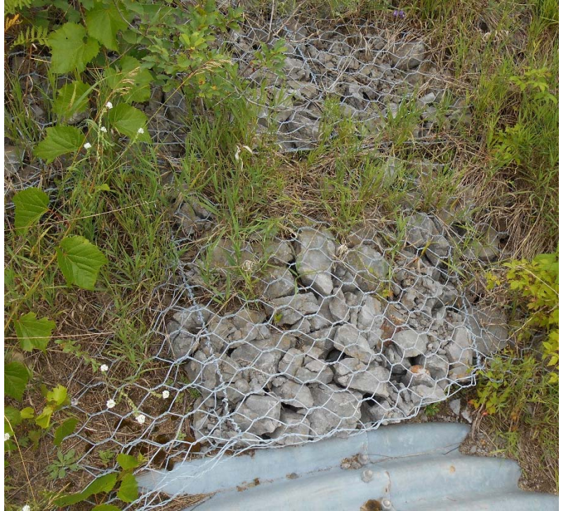
Overtop looking down on inlet showing condition of gabions
