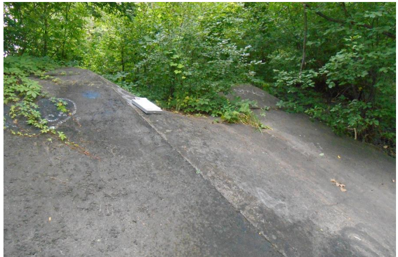
Concrete lining of creek bank, located along the north creek bank north of inlet
