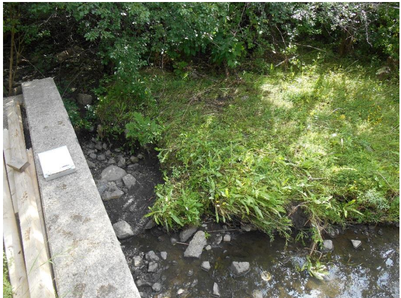
South outlet, note the erosion of the bank in front of the culvert
