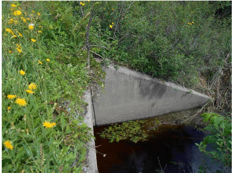
Condition of north tapered portal wall at inlet
