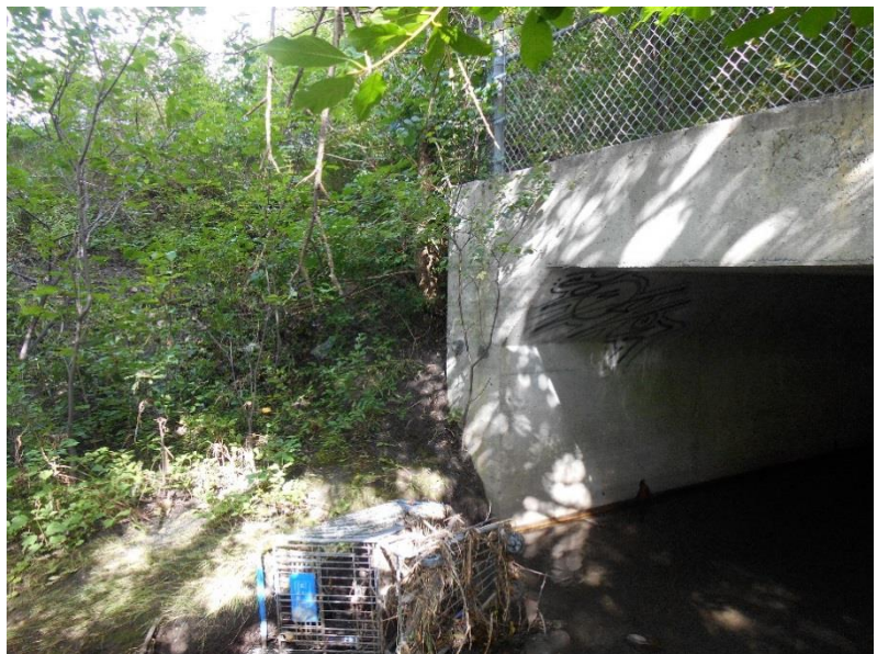
South outlet, note erosion of slope
