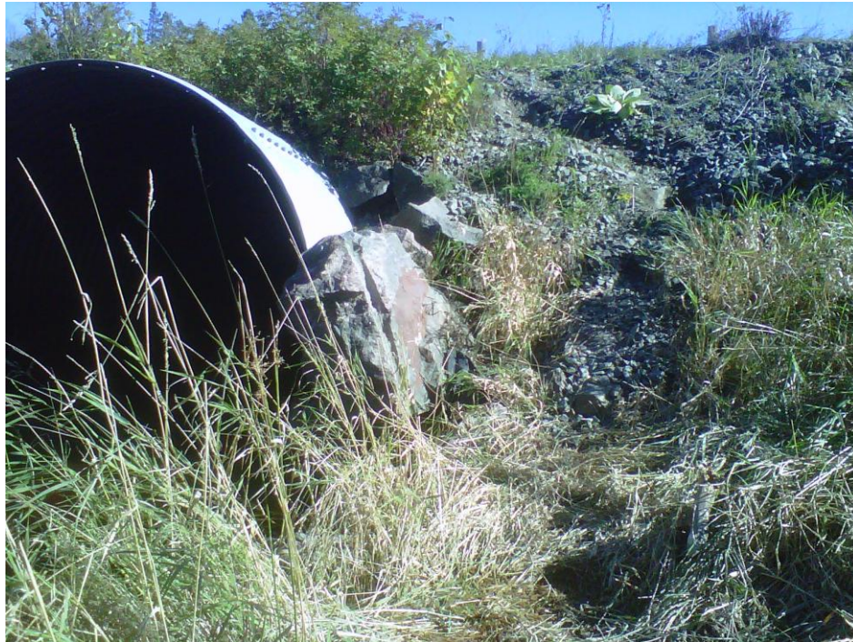
Figure 2.1 Corrugated Steel Pipe (CSP) culvert (looking south)
