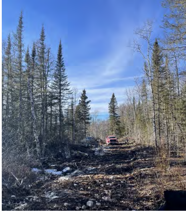
Photo 7: Section HF4 looking west along CL near Sta 12+200, photo taken March 5, 2024
