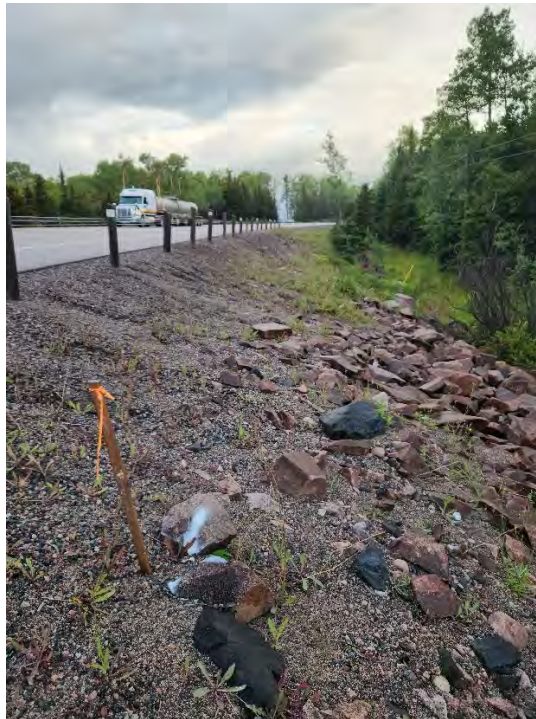
Photo 12: Section DC1 looking west along Highway 17 near Sta 12+660, photo taken August 17, 2023
