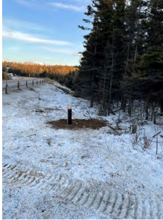
Photo 11: Borehole DC1-04 near Sta 12+500 looking east, photo taken March 1, 2024
