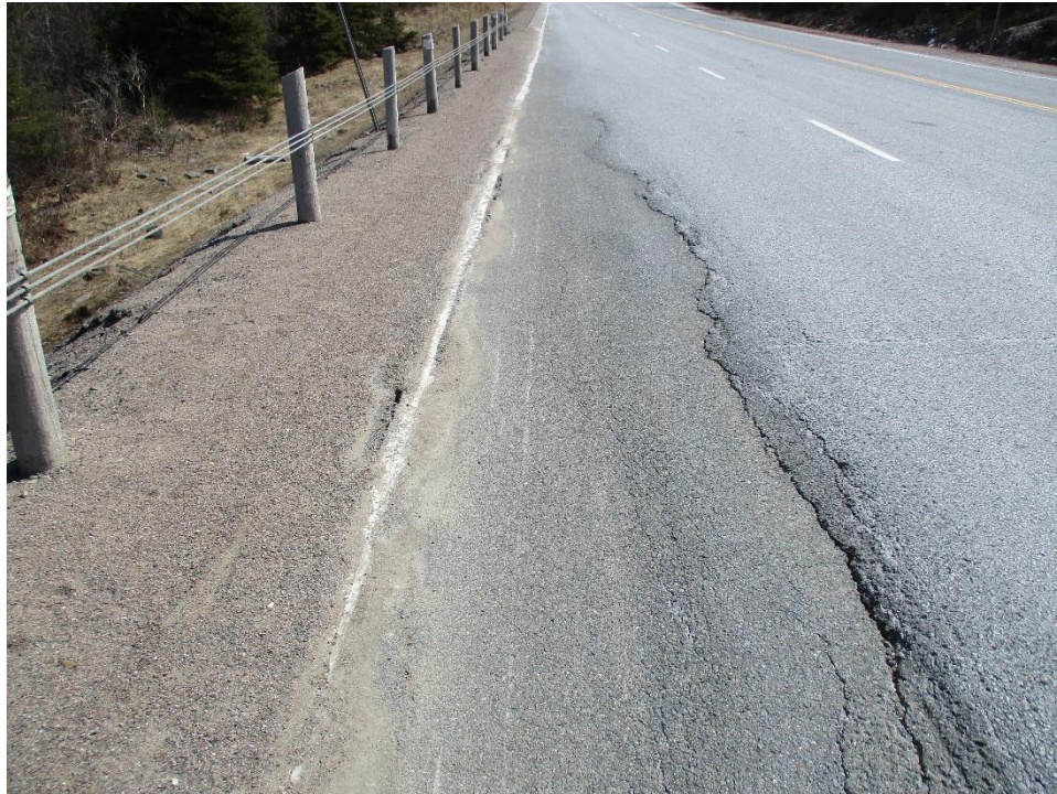
Photograph 1: Area of instability. Outside westbound lane looking east [taken May 2021, Credit MTO]
