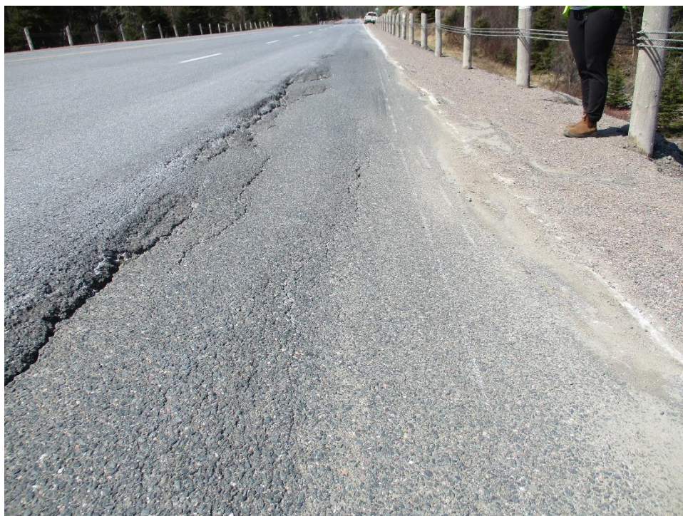
Photograph 1: Area of instability. Outside westbound lane looking west [taken May 2021, Credit MTO]
