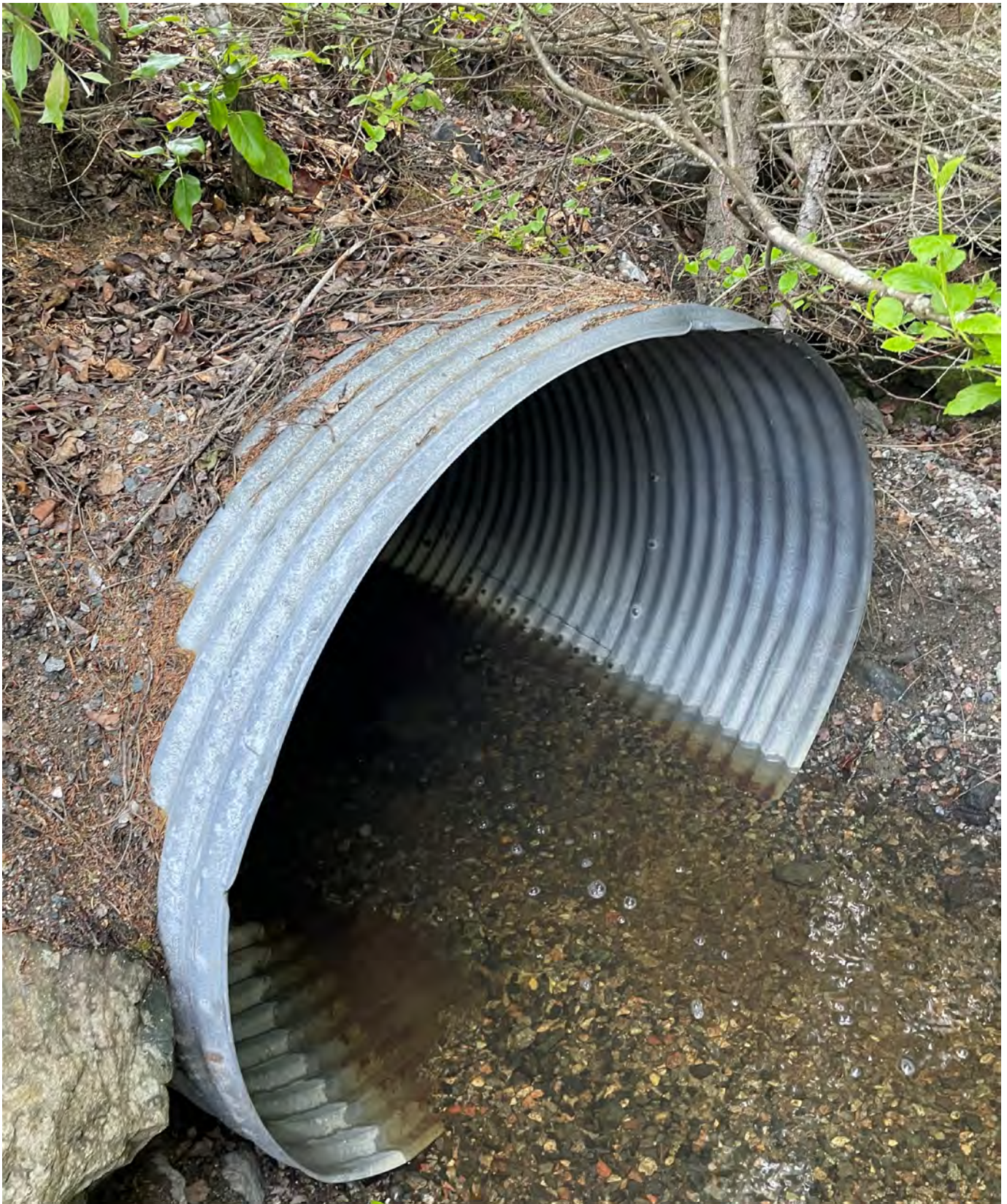
Photograph #12 – CSP extension at culvert outlet. (June 2024)
