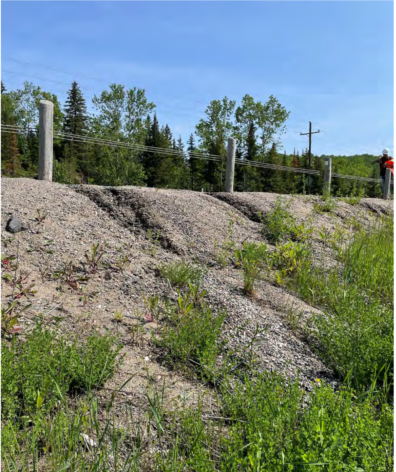
Photograph #10 – Surficial erosion at the crest of embankment beyond the south shoulder. (June 2024)
