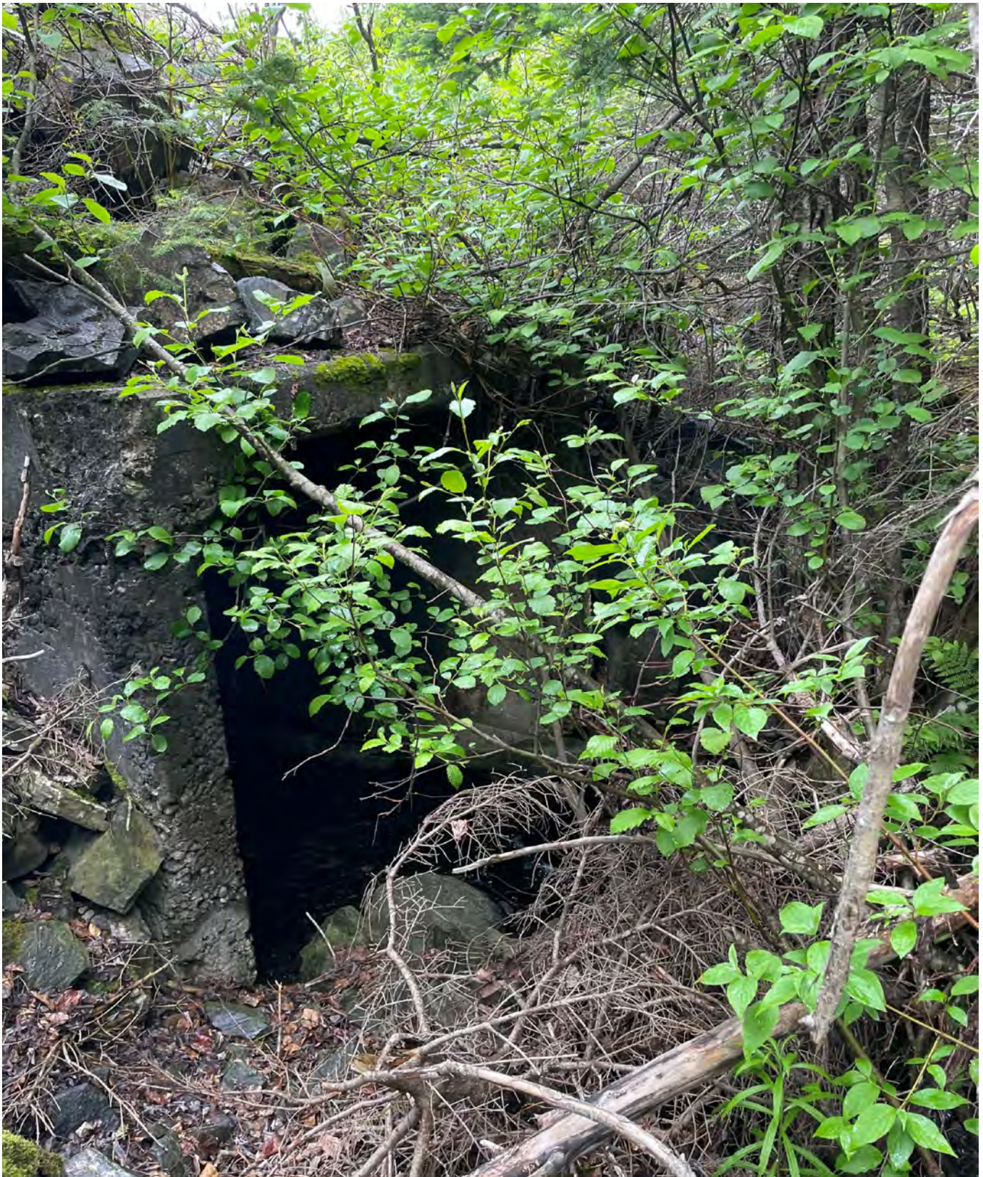
Photograph #5 – Culvert inlet obstructed with vegetation and other debris. (June 2024)
