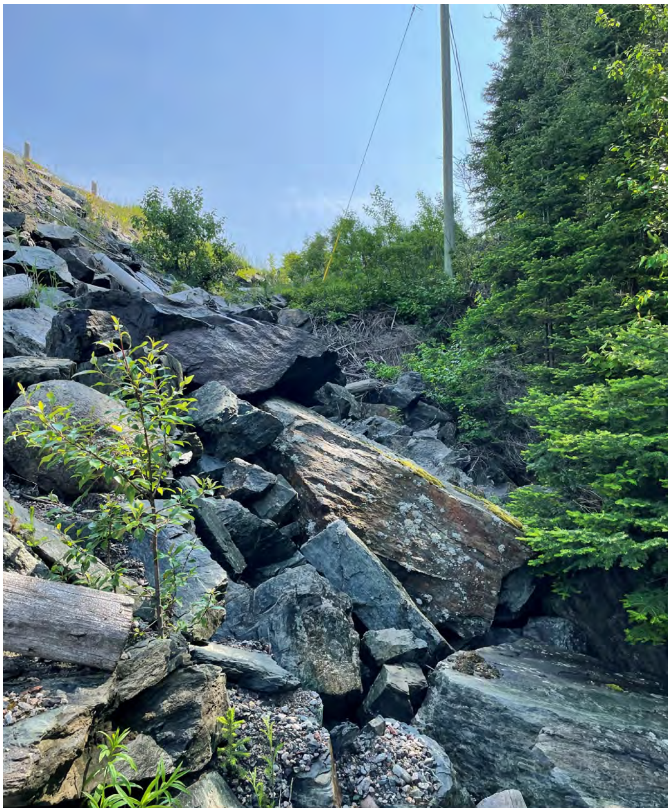
Photograph #8 – Rock fill on steep south embankment slope looking east. (June 2024)
