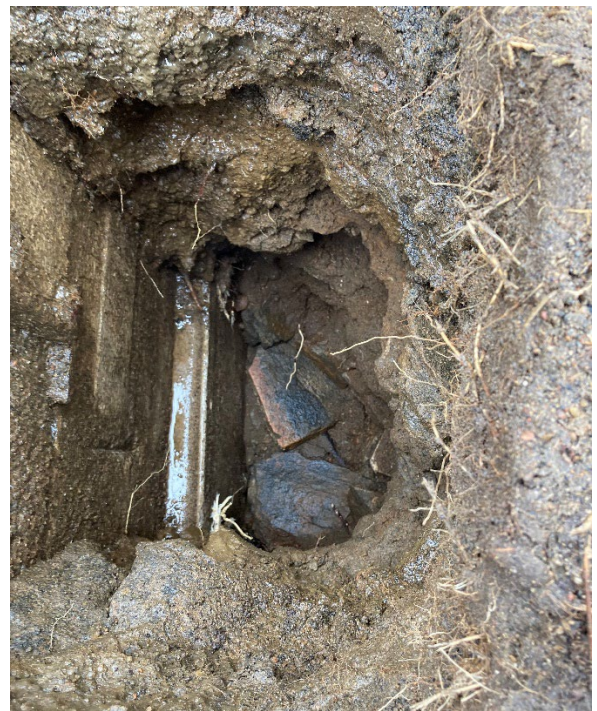
Looking Downhole at Exposed I-Beam and Rockfill
