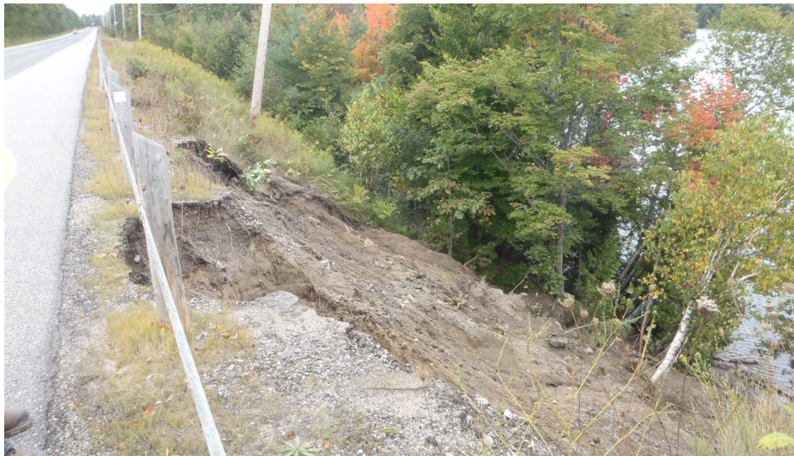
Photograph 2: Highway 7289 and east slope showing failure (looking north) [taken Sept. 2014]
