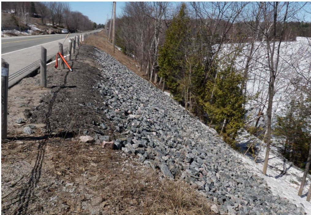
Photograph 4: New slope treatment near Sta. 11+770 (looking north) [taken Apr. 2015]
