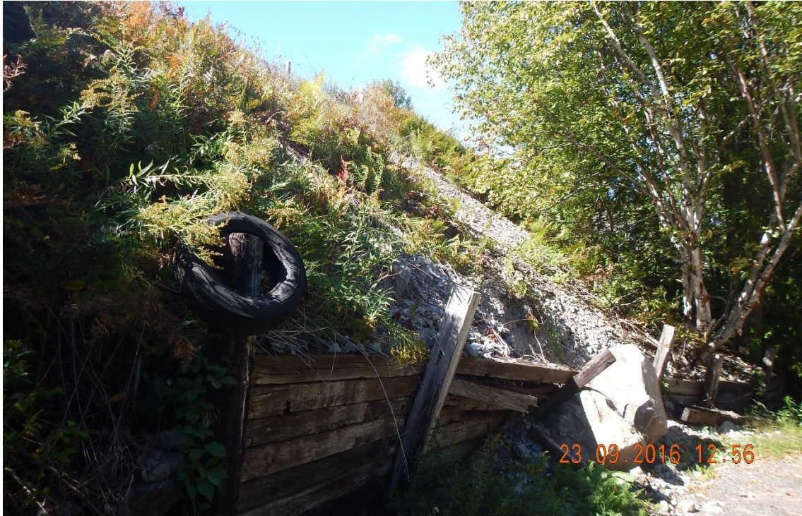
Photograph 5: Existing Timber Retaining Wall near Sta. 11+475 (looking north) [taken Sept. 2016]
