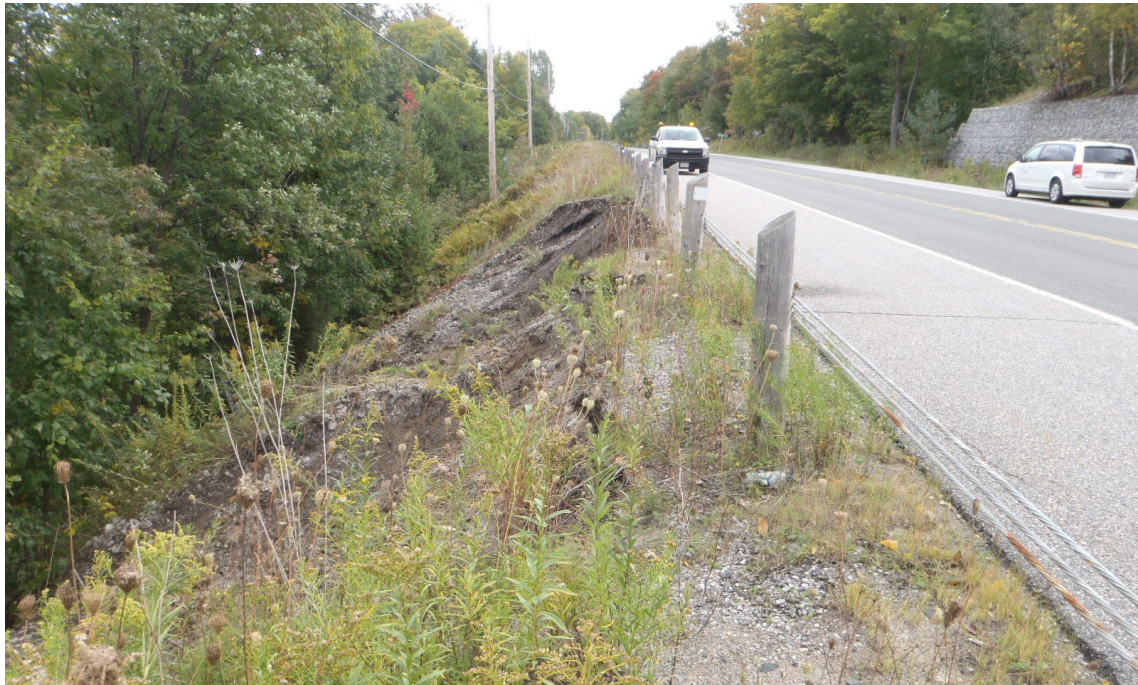
Photograph 1: Highway 7289 and east slope showing failure near Sta. 11+510 (looking south) [taken Sept. 2014]
