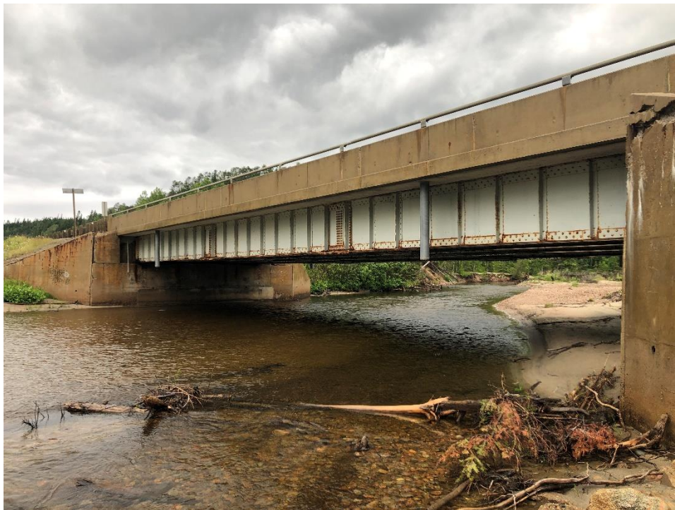
Photograph 10: Deposited sand and tree debris near the south abutment [taken August 2022]
