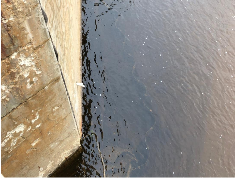
Photograph 9: Sheet piles below water at the east side of the north abutment [taken August 2022]
