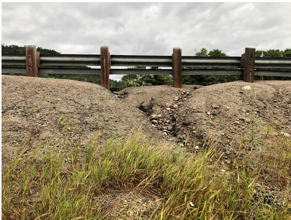
Photograph 8: Erosion at the south abutment's west side slope [taken August 2022]
