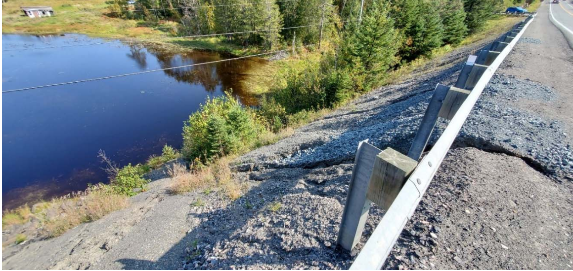
Photo 1: Looking northeast along north embankment slope. Granular slope, erosion gullies, localized crushed rock repairs, vegetation at the east end of embankment and body of water at embankment toe. Photo taken near location of culvert crossing. [taken September 2020]
