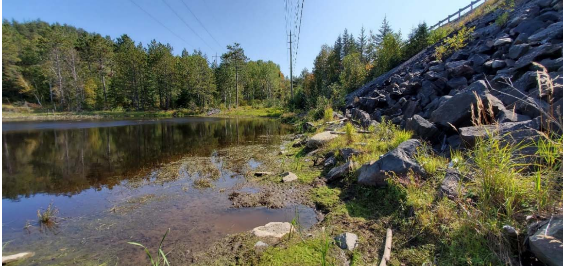
Photo 3: Looking eastward along north embankment toe. Water at toe of rock lined slope. Utility lines overhead and Buried Bell utility. [taken September 2020]
