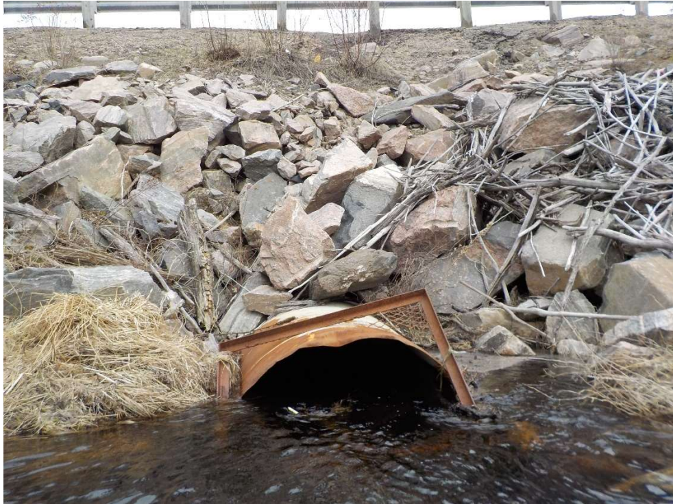
Photo 1: Culvert inlet (taken by MPCE) [Summer 2023]
