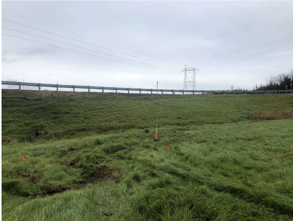
Photo 2. Looking northeast toward W-N/S ramp from Borehole 20-02 [Oct. 2020].
