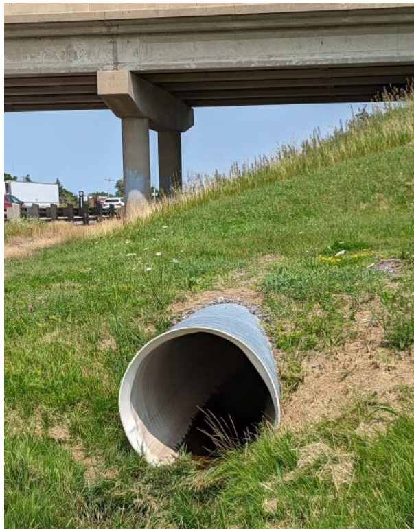
Photograph 5: Existing ditchline culvert under the proposed south foreslope footprint typical; July 10, 2023
