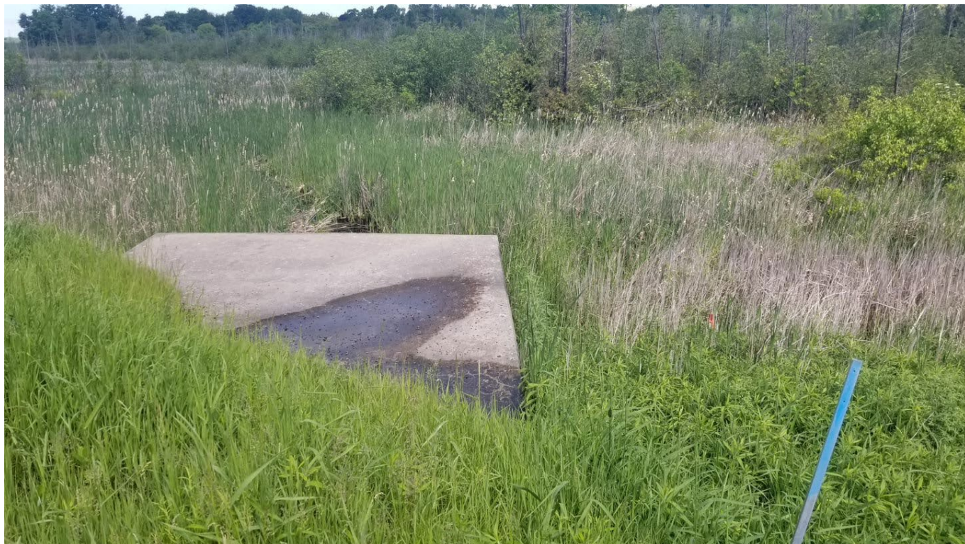
Photograph 3: Existing Culvert Outlet (North End), Facing North
