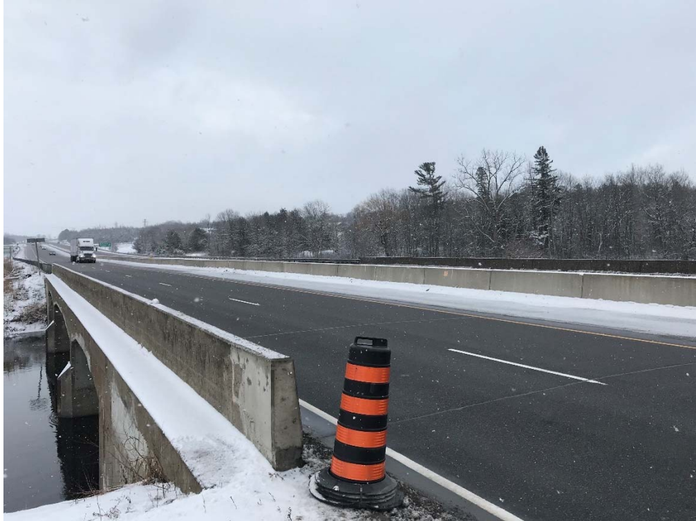
Photo 3. Looking south-east along Highway 401 [December 2019]
