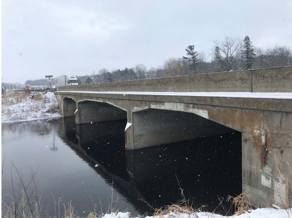
Photo 1. Looking south-east at north bridge profile [December 2019]
