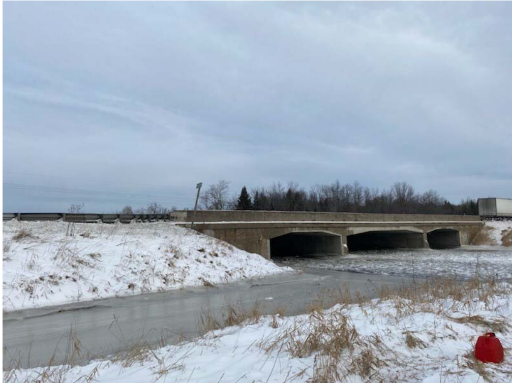
Photo 4. Looking north-east at the south bridge profile [January 2020]
