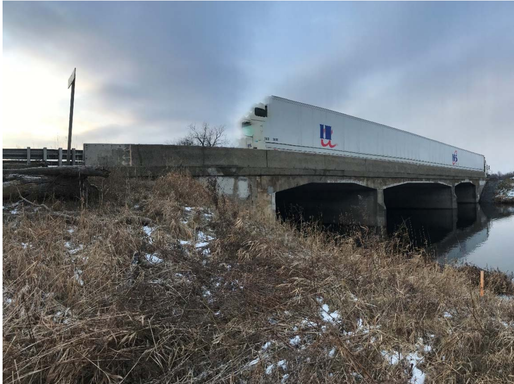
Photo 2. Looking south-west at north bridge profile [January 2020]
