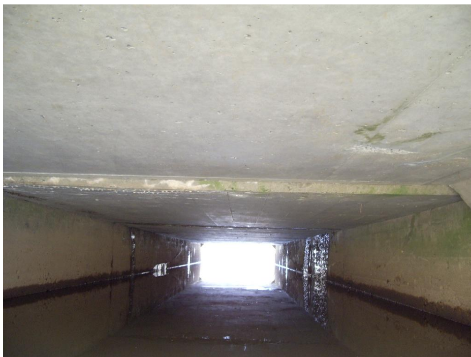
Photograph 3 - Interior of culvert, looking downstream from inlet (north end). Leakage is evident near centre of culvert.
