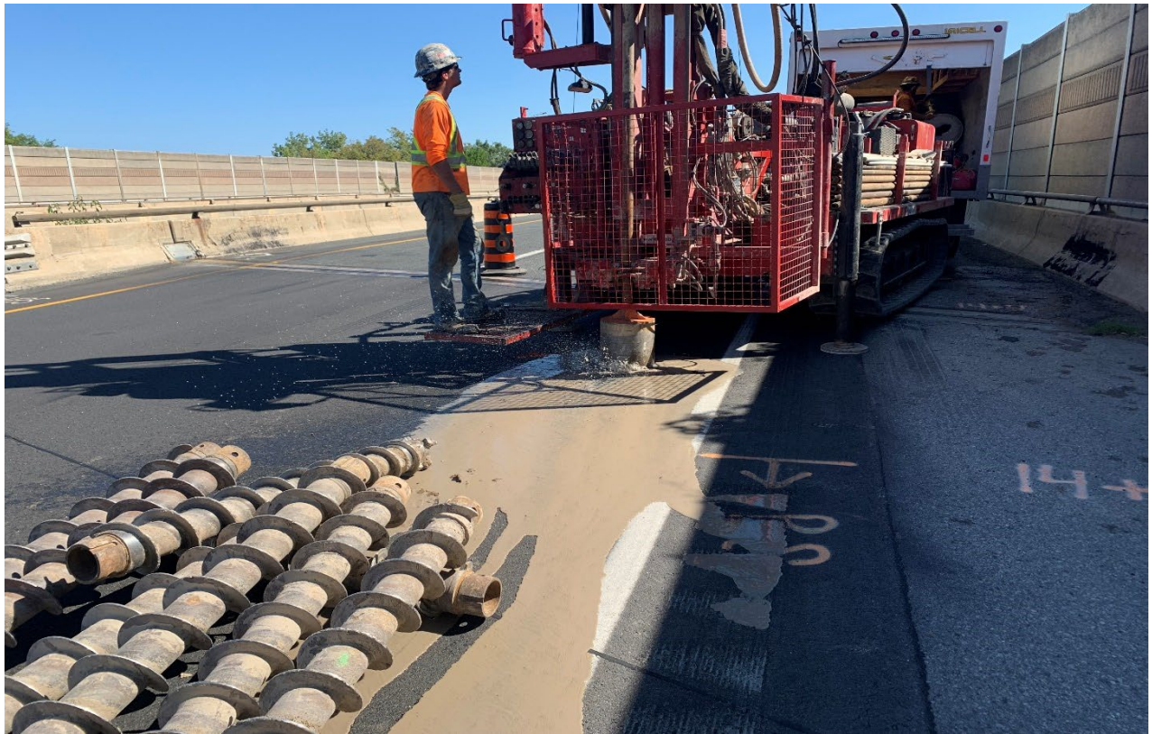
Photograph 1 – Drilling operations at Borehole, BH2-22 – Highway 402 Eastbound Lane
