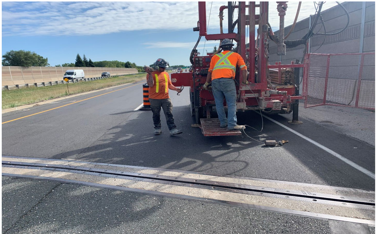
Photograph 4 – Drilling set up at Borehole, BH1-22 – Highway 402 Westbound Lane
